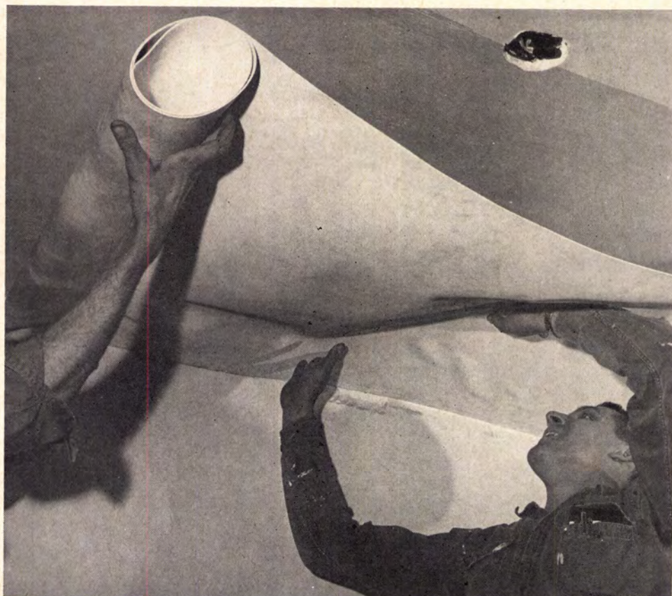
MASTIC COATING bonds radiant vinyl to ceiling. Bubbles are smoothed out with long-handled roller.
