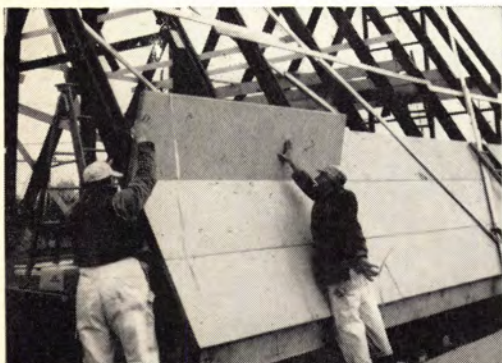
T & G panels, 2' x 8', serve as decking and side-wall for this A-frame with 48" o.c. spans. Interior surface can be factory-coated in white, beige or special color to order—with vapor barrier and vinyl film or white kraft surface.
