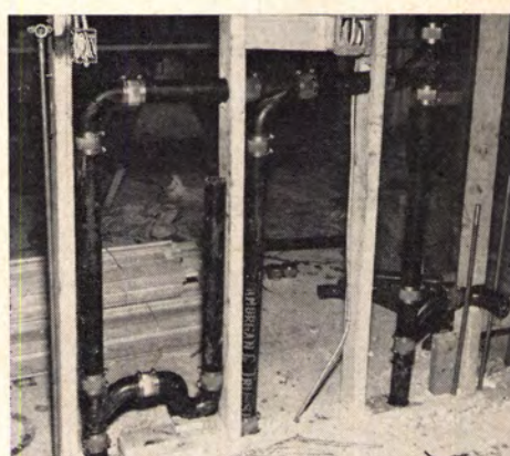
WASTE SYSTEM of sleeve-joined pipe is attempt to make plumbing layout more flexible.
