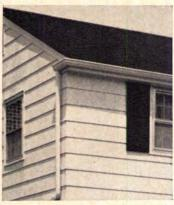
Factory-finished siding is primed baseboard with a vinyl copolymer finish. According to the manufacturer, the material is resistant to checking, peeling and weathering. A ten year written guarantee is included. Insulite, International Falls, Minn.
