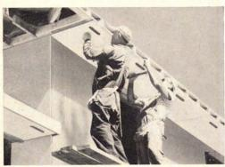
"Soffitsote" panels in 10 sizes are factory-primed and fitted with 8-mesh, factory-cut vents, 48" o.c. Meets FHA requirement for roof area ventilation.
