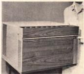
Wood-faced air conditioner has all controls hidden except for the on-off button. Regulation of air circulation and cooling is automatic. Manufacturer says units are up to 56% quieter than others tested. Amana Refrigeration, Amana, Iowa.
