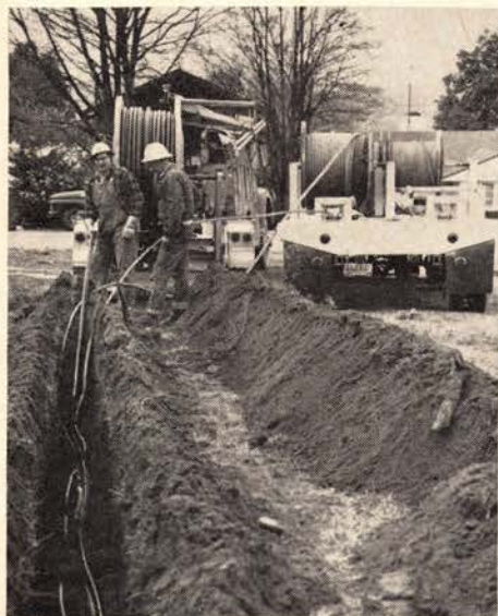
JOINT BURIAL reduces per-lot costs of underground wiring. Washington state changed code to allow phone and power cables in the same ditch.
