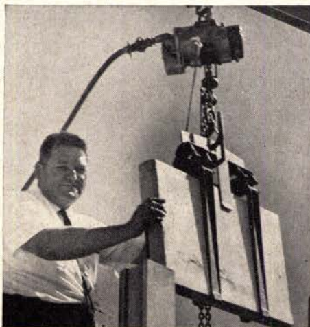
7. PRECAST PANEL , stacked between column grooves, measures 18"x36"x3" and weighs 170 lbs.
