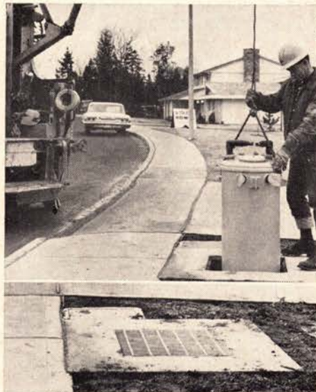
HIDDEN TRANSFORMER is put underground by Puget Sound Power workman (top), leaving flush grate (bottom) as only trace of electric system.
