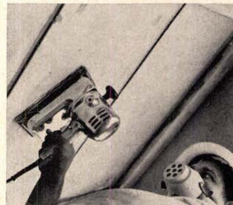
10. FINISH SURFACE is structural concrete buffed up by sander (after defects are patched).
