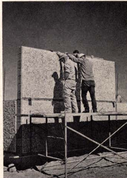
AGGREGATE FACINGS are easily applied to block panels because work can be laid flat.
