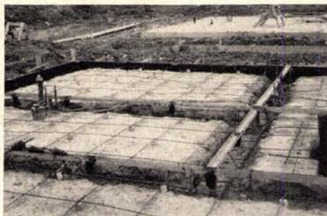
1. POURED FOUNDATION , containing plumbing hookup, ties reinforced slab to column footings.
