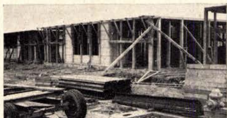
9. POURED ROOF takes major formwork but eliminates big slab and heavy lifting equipment.
