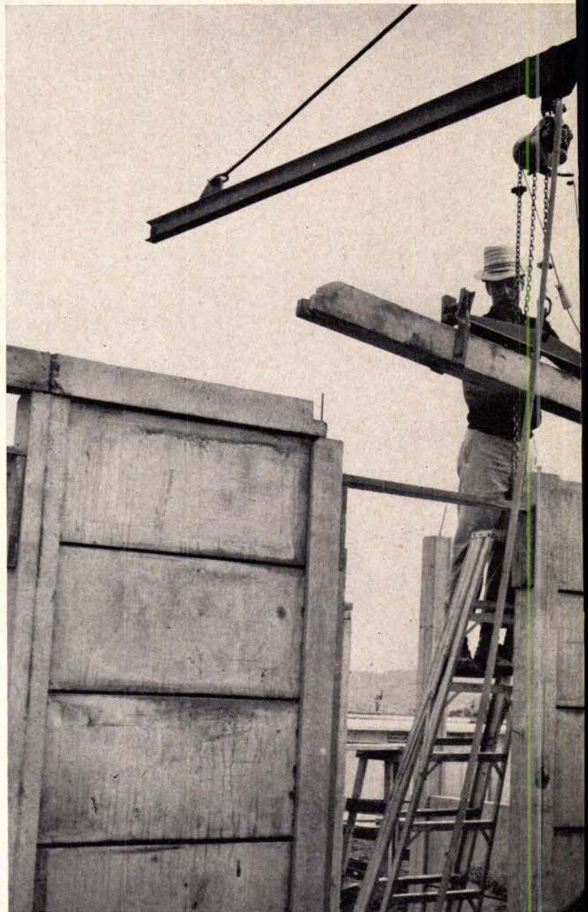
SHORT BEAMS cap small-component wall, tying together columns and providing bearing plate for poured roof. All precast parts are handled by small air hoist.
