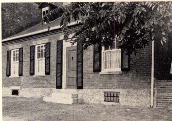
AFTER: Sandblasting to remove paint was part of $5,000 fix-up cost.
