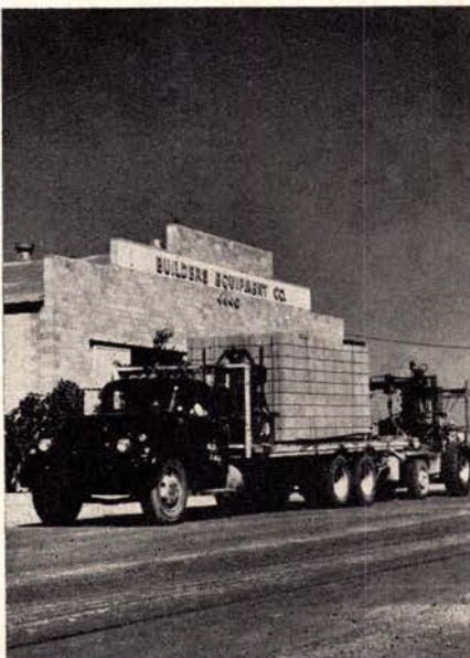
48-HOUR DELIVERY of block panels—ten per truck—is made possible by fast-set mortar.
