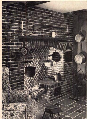
Brick substitute is installed with a mastic that looks like cement when dry. Waterproof bricks are available in four color-fast shades for indoor or outdoor use. Rough and smooth finishes are offered. Dacor Mfg., Worcester, Mass. Circle 201 on Reader Service card.
