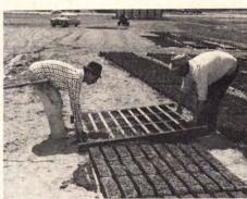
4. Forms are removed after partial drying.
