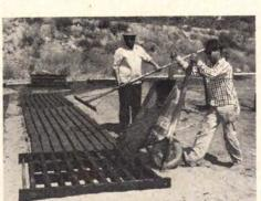
3. Mixture is poured into open wood forms.
