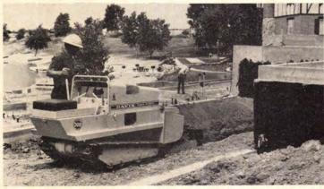
Wide-track trencher has a flotation of 2.69 psi in mucky or sandy areas. Three track sizes available: self-cleaning 8" and 10" cleat tracks and 10" street tracks. A variety of attachments are also offered. Davis, Wichita, Kan. Circle 233 on Reader Service card.
