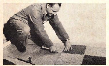
**Interlocking rug-tiles** form a continuous surface and do not require adhesives. The 12" square polystyrene tiles are covered by seven carpet grades, which are available in 40 colors. Roxbury Carpet, Saxonville, Mass. Circle 119 on Reader Service card.
