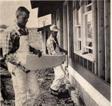
**Rigid vinyl plastic siding** will not show abrasions, mars, scars or scratches and won't peel, corrode or blister, says the manufacturer. Installation is with nails through insulation board. Comes in 12'6" length. Mastic Corp., South Bend. Circle 173 on Reader Service card.
