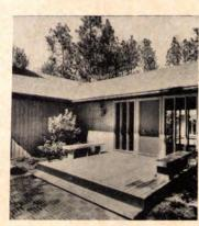
Rough sawn siding has a stain-type finish that combines preservatives, water repellents and pigment, Siding is durable and easy and inexpensive to apply, according to the manufacturer. Southern Pine Assn., New Orleans, La.
