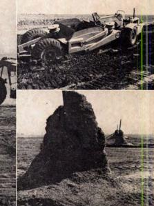
and are easier to pull out. When existing land is cut, columns of earth are left to mark original grade (bottom right).
