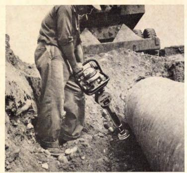
**Lightweight rammer,** Model GVR 30, delivers up to 1,050 blows a minute. The portable unit has an air-cooled, 1-cylinder, 2-cycle gasoline motor. Soil layers up to 10" in depth can be compacted with this machine. Wacker, Hartford, Wis. Circle 230 on Reader Service card.
