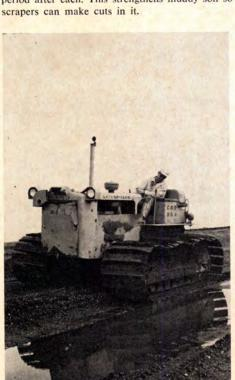
5. Crawler tractor with extra-wide track shoes squeezes water from newly placed hydraulic fill before big scrapers move in for final grading.
