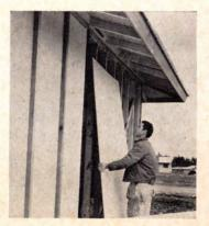
Pre-primed panels have a light gray acrylic latex paint baked on. The surface is said to have superior paint-holding properties and resistance to chalking and deterioration. One coat of finish paint is required. St. Regis Paper, Tacoma.
