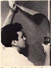
Sound-deadening cork can be installed underneath flooring or behind gypsum wall board. It is offered in 4' wide and 100' long rolls or in sheets. It can be stapled, nailed or laminated into place. Dodge Cork, Lancaster,
