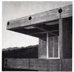
CABLE TERMINALS are left exposed at deck edge for tensioning about two days after pour,
