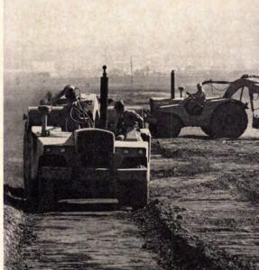
2. Small 8-cu.-yd. scrapers are used for leveling the soft soil prior to filling. They get mired down less often than 20-cu.-yd. machines (top right)
