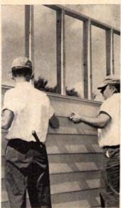
Aluminum panel is installed directly over studs. Material consists of an enameled aluminum panel, polystyrene insulating foam and a heavy covering of bonded aluminum foil. Panels are said to be maintenance free. Alsco, Akron, Ohio.
