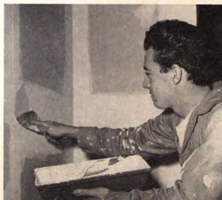
TWO POINT-UPS —one after sanding ( above ) and one after paint-priming—help insure that even smallest defects won't be overlooked.
