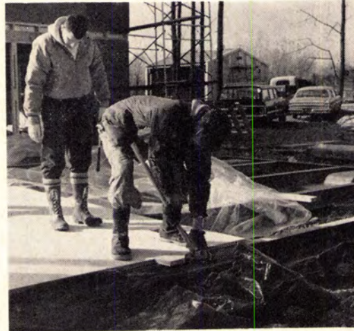
PLYWOOD SUBFLOOR is fastened directly to I-beams. A heavier floor panel may permit 5' joist spacing.
