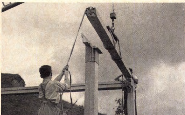
FRAMING for panels is concrete columns and beams poured in plastic forms.
