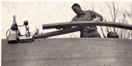
HEAT WELD by machine bonds boards together.
