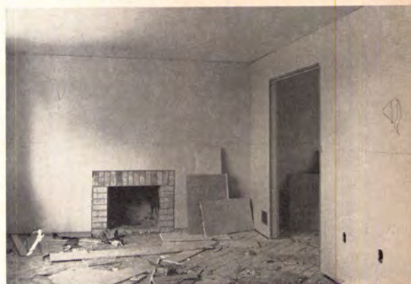
LONG SHEETS minimize drywall cracks by minimizing seams. Henry stocks the longest sheets he can buy (14'), uses them wherever possible.
