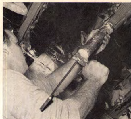
MASTIC-PLUS-NAILS is Henry's double-safe method for hanging drywall. It minimizes cracks and nail pops, giving him a low callback rate.
