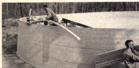
FOAM BOARDS are laid up to construct dome.
