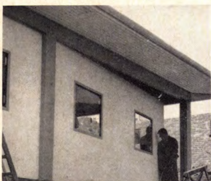
PANELS are fastened against column flanges by plastic-covered wood trim.
