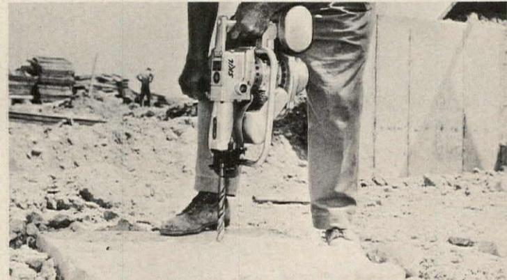
**Gasoline-driven rotating hammer** bores holes up to 2". An all-attitude carburetor allows full-speed operation in any position, so it can work upside down for jobs on ceilings and horizontally for boring walls. Skil, Chicago. *Circle 261 on Reader Service card*
