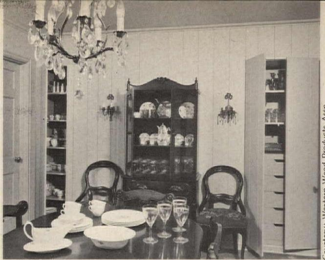
**TWIN CHINA CLOSETS**, with adjustable shelving, are set into wall of solid board paneling. Lower half of one closet has drawers for linen and silver. Doors have touch latches.
