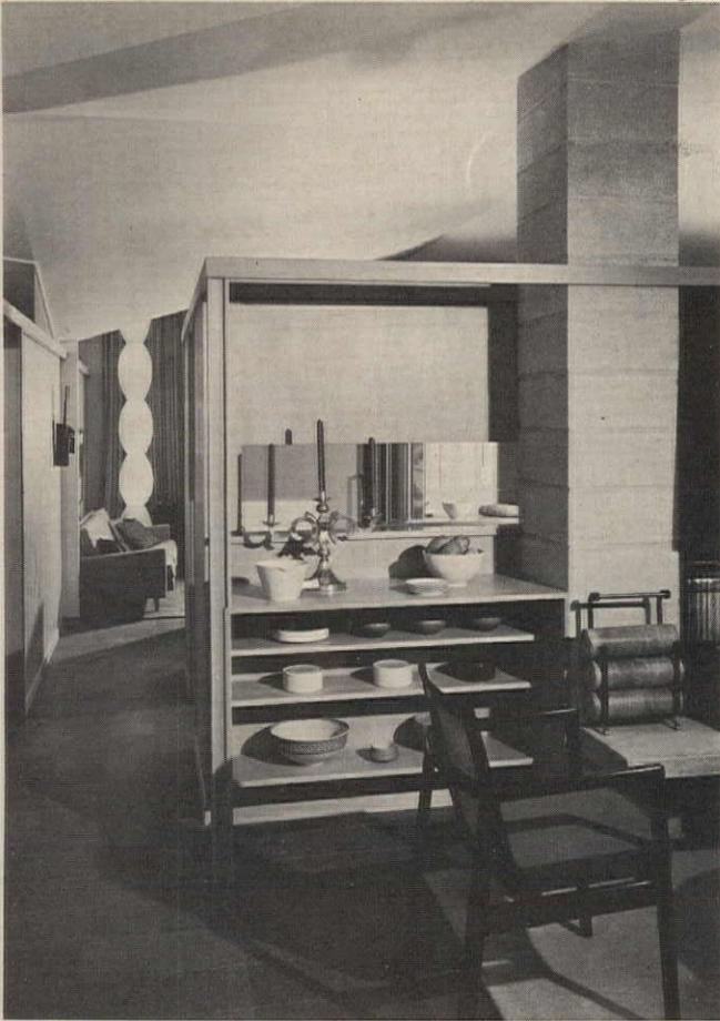
**OPEN CHINA SHELVES** are built into dividing wall between kitchen and dining room, in foreground, and anchored to chimney wall. Top shelf serves as pass-through counter.
