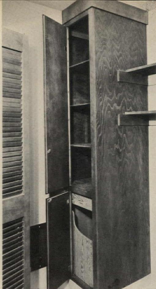
**LAUNDRY PASS-THROUGH** in Stephens' model is a ceiling-high linen closet built into washer-dryer room (*left photo*) with doors
