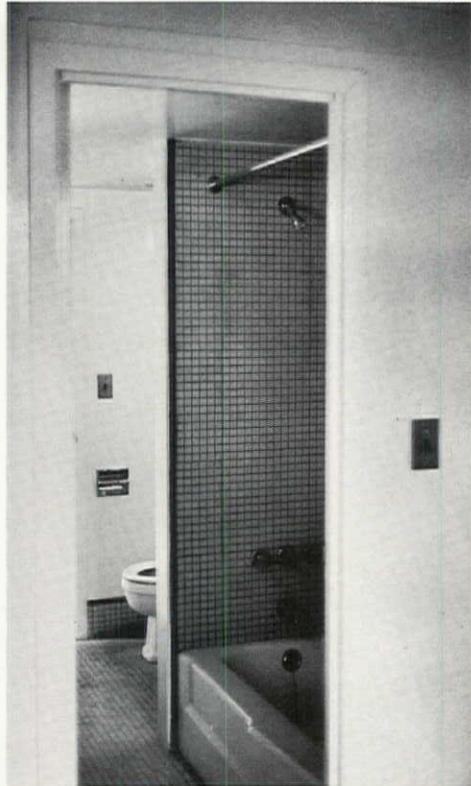
**IN-PLACE CORE**, heart of rehabilitation system being tested in New York City tenement, has kitchen (left) backed up to bath (right). Note fuse box and heating vents on core wall.
