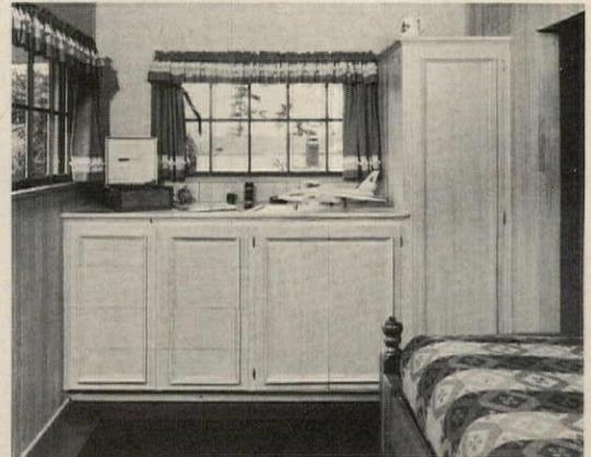
**UNDER-WINDOW STORAGE** puts drawer and hanging space in below-grade area of a split-level house. This unit has full-length closet, shirt-and-slack cupboard, and double bank of 18"-wide drawers. Applied molding strips give paneled effect.
