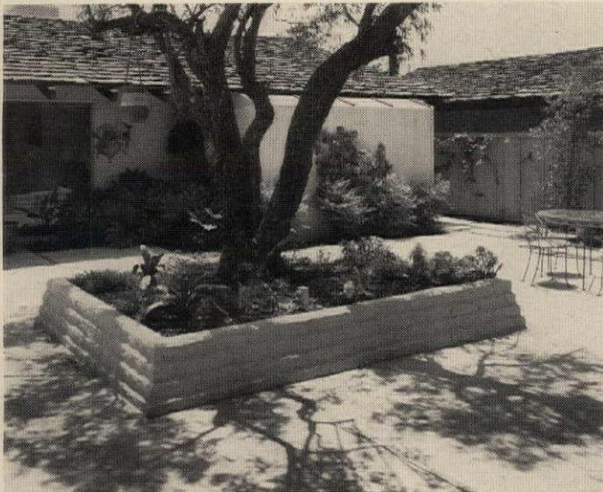
**New-style concrete masonry—simple way to give patios extra charm.** Decorative Concrete makes this patio a "people pleaser." Central planter is of painted concrete slump block. Flatwork surfacing is lightly textured. Decorative Concrete can be adapted to any building budget.
