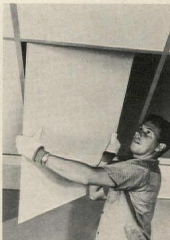
**Radiant heating panels** for use in suspended ceiling grids come in two models: 1) a 750-watt unit with three to six heaters per control and a 2,560 Btuh rating; 2) a 500-watt model with four to eight heaters. Litecontrol, Watertown, Mass.
