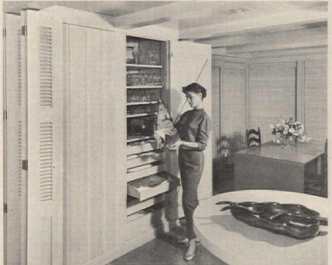
**BUILT-IN SIDEBOARD** includes shelves for dinnerware, drawers for linens. Doors have spring latches; Z-shaped braces and hardware are concealed on inner sides of doors.
