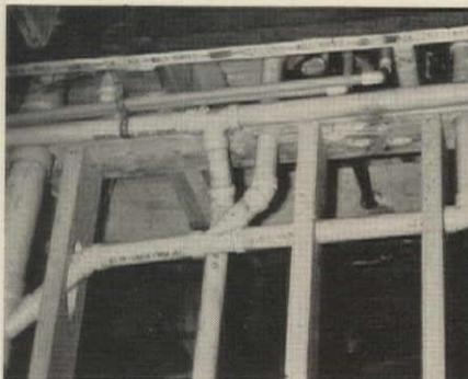
5. Installation was remarkably easy in tight, hard-to-get-at places because solvent cemented joints eliminated threading and soldering.
