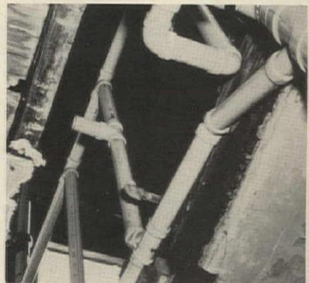
6. Maximum safety was achieved because torches were not required for installation; this was especially important in confined, "tinder-dry" construction.
