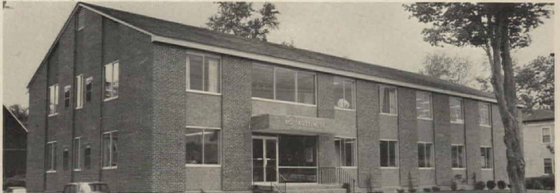
**TRUSS-ROOF OFFICE BUILDING** with precast floors, brick-veneered block walls and 12,000 rentable sq. ft.
