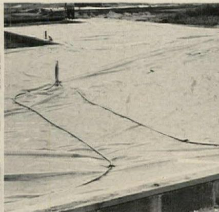
second man anchors tube to compacted soil. Boiler connection (*center*) will be made above slab. Absence of registers speeds pouring (*right*).
