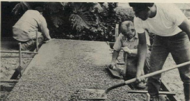
3. Colorful aggregate of uniform size (¼- to ½-inch on this job) is seeded from shovel. In background two finishers have already begun tamping in aggregate with wooden hand floats.
