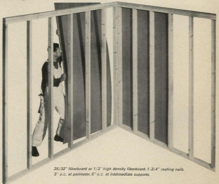
*25/32" fiberboard or 1/2" high density fiberboard, 1-3/4" roofing nails
