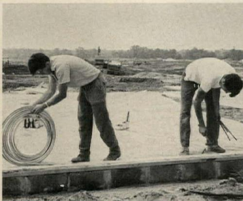
**UNDER-SLAB TUBING** is installed by two-man crew. First man unrolls a one-house supply—contained in a single coil, which eliminates joints—while
