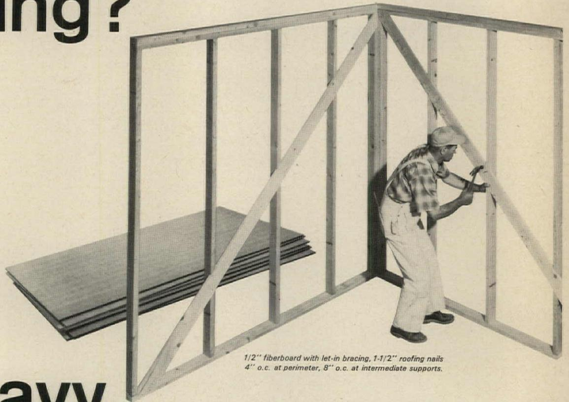
*1/2" fiberboard with let-in bracing, 1-1/2" roofing nails
