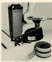
Automatic nailer—the first to drive nails in the 1¼" to 1½" range—takes a coil-type 300-nail cartridge. Nails feed automatically as fast as nailer is operated —up to 280 nails per minute. Weight: 7½ lbs. Duo-Fast Fastener, Franklin Park, Ill.
