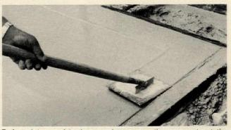
5. An edging tool is then used to secure the aggregate at the edges. This is final step before concrete sets up enough to begin the hosing and brushing operations.
