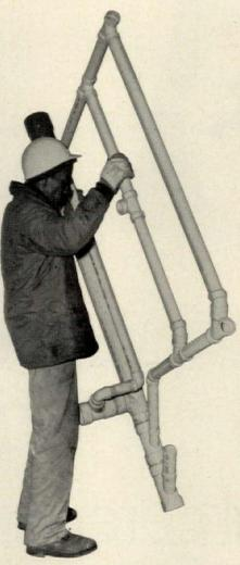
**4.** PVC pipe is lightweight and easy to install through and around the existing framing. It can readily be preassembled.
