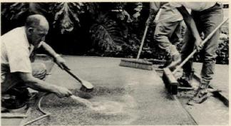
Medium-bristle push brooms are used for major brushing. The man with the hose touches up areas missed by the large brooms. This is the final step in producing the exposed aggregate finish.
