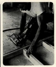
1. Wall assemblies are fast with a CN-137 Nailer driving coated 16d sinkers.
