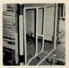
7. The simple method of joining PVC and CPVC piping is highly efficient on one job only four leaks out of 5000 joints. And they were easily corrected. Expansion joints, shown here, were used between floors and performed equally well.
