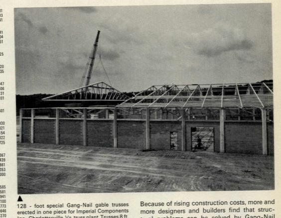
128 - foot special Gang-Nail gable trusses erected in one piece for Imperial Components Inc., Charlottesville, Va. truss plant. Trusses 8 ft. OC for 40 psf.-Stainback & Scribner, AIA.
