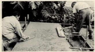
As aggregate embedment is completed along the edges one finisher uses a wood bull float to cover the center. Floating is continued until all aggregate is completely embedded.
