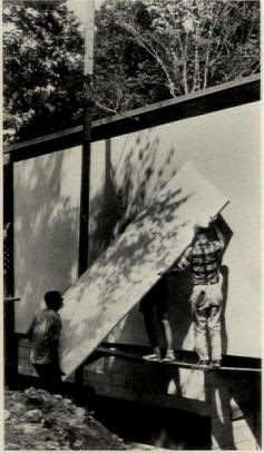
**EXTERIOR INSTALLATION** is easily handled by workmen. Material weighs only 2 lbs. per sq. ft.
