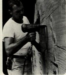
**3.** Sheathing holds tighter with 2" staples driven by a Duo-Fast Staple Nailer.
