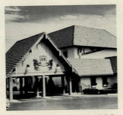
Schneithorst's Bavarian Inn. Gang-Nail flat roof trusses for mansard span 47 ft. and are 13½ ft. high. Trusses fabricated by Wood Tech Corp., Kirkwood, Mo.-Robert Elkington, AIA.
