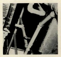
6. Maximum safety was achieved because torches were not required for installation; this was especially important in confined, "tinder-dry" construction.
