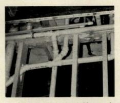
5. Installation was remarkably easy in tight, hard-to-get-at places because solvent cemented joints eliminated threading and soldering.
