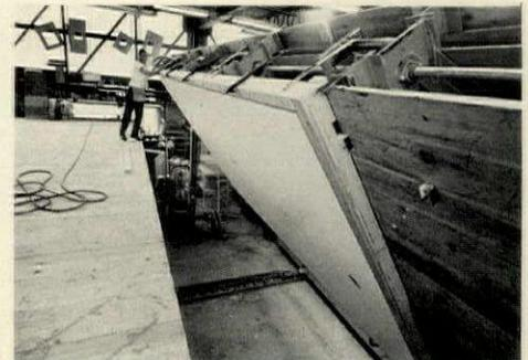
**CEILING UNIT** is turned over after being fabricated upside-down on platform above assembly line. Unit is then lowered onto module.
