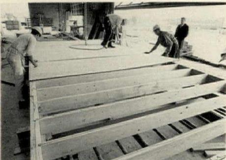
**FLOOR DECK** is sheathed after being assembled upside-down to assure precise joist alignment. Glue-nail fastening guarantees structural rigidity.
