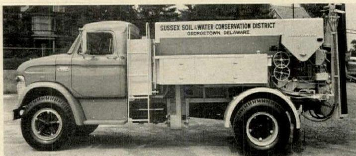
**SMALL MODEL** of 4-cu.-yd. capacity is powered by truck engine. Pouring rate is one cubic yard per two to four minutes, depending on type of mix.
