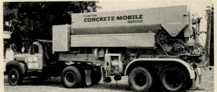
**LARGE MODEL** of 10-cu.-yd. capacity is mounted on a trailer and powered by auxiliary engine. Mixer operators are trained at manufacturer's factory.
