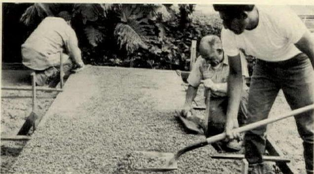
3. Colorful aggregate of uniform size (1/4- to 1/2-inch on this job) is seeded from shovel. In background two finishers have already begun tamping in aggregate with wooden hand floats.
