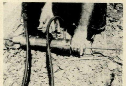
**HYDRAULIC JACK** pulls tendon to specified final tension by ramming anchor chuck into place.
