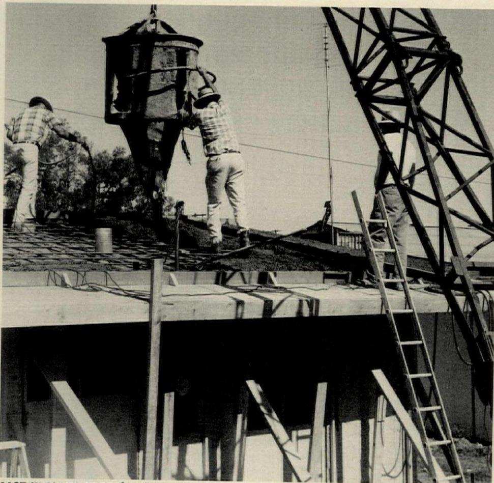
**CAST-IN-PLACE ROOF** for all-concrete house ties together tilt-up walls by means of overlapping reinforcing bars (see also drawing at upper right). Roof pour for 768-sq.-ft. house takes three hours.
