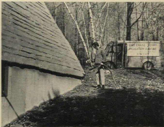
keeping the two ingredients proportioned right. I've seen cases where the insulation never hardened or where it didn't bond to the substrate because the mixture was wrong."
