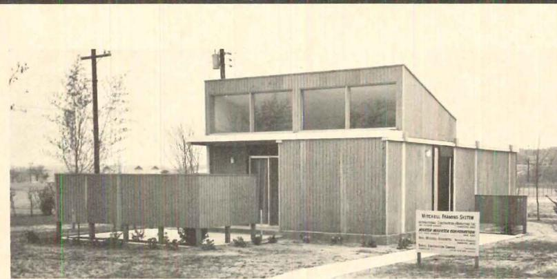
**PRECAST CONCRETE FRAME WITH CURTAIN WALLS** encloses this 654 sq. ft. house, which costs \$7,000 and takes about four weeks to build.
