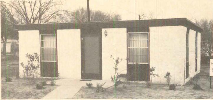
**CONCRETE SACKS PINNED TOGETHER BY RODS** form the exterior walls of this 676-sq.-ft. house with two bedrooms and one bath.
