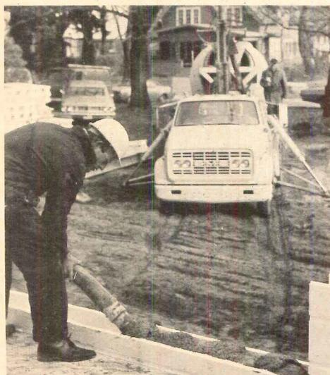
**PUMPED CONCRETE**, delivered through hose on truck boom, fills upper courses of plastic forms.
