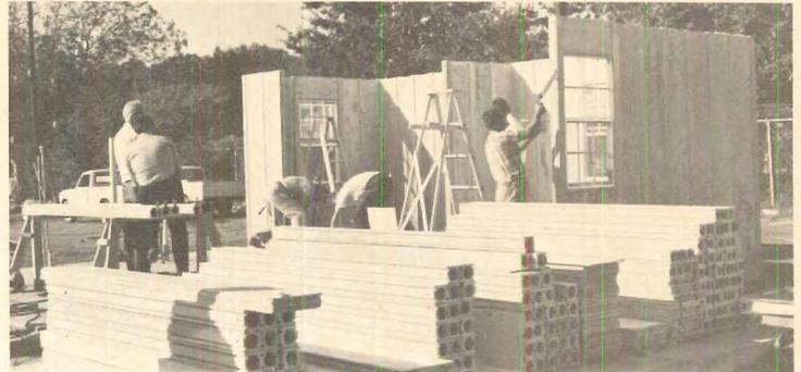
panels—one for each side of the wall—are inserted between each set of posts, and the space between them is filled with 2"-thick fiberglass batts (right).
