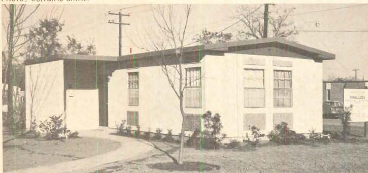
**PRECAST CONCRETE PANELS IN ALUMINUM FRAMES** are the exterior walls of this four-bedroom, one-bath house.
