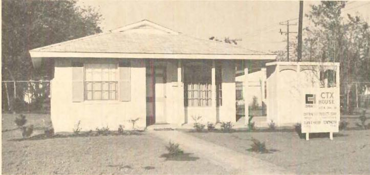
**ASBESTOS-CEMENT EXTRUSIONS FOR WALLS** set this 591-
