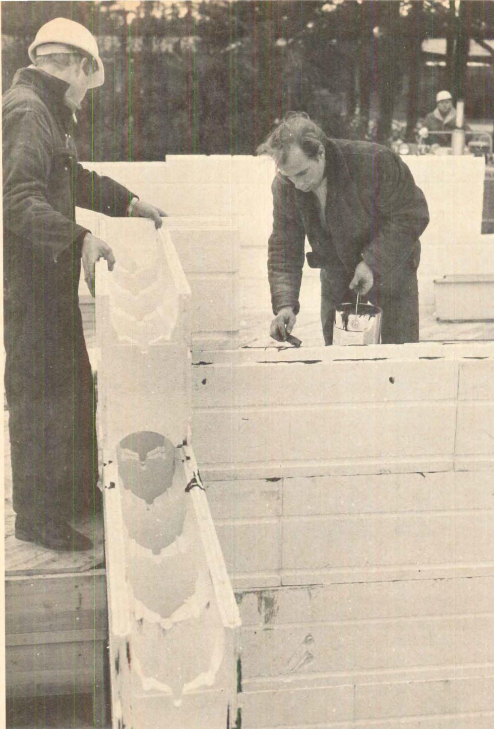
**POLYSTYRENE FORM ASSEMBLY** is simplified by T&G edges, which are glued together, and molded reinforcing-rod channels. No special skills are required, but vertical cores must be aligned precisely.
