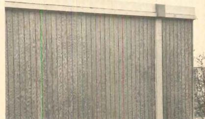
Framing components—posts, lintels and beams (*photo, right*)—can be cast at the site or in a factory. They are made with lightweight concrete designed especially for the system by the engineer—Neal Mitchell Associates of Cambridge, Mass. But they are heavy enough to permit future expansion of the house upward as well as sideways. The foundation is grade beams on drilled piers.
