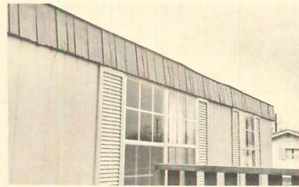
While the dimensions and floor plan resemble those of a standard mobile home, the construction is somewhat heavier. Exterior walls, for example, are framed with 2x4s clad with 1/2" firecode sheathing under prefinished aluminum siding. But interior partitions are made of 2x2s clad with 1/4" Lauan plywood. The floor is framed with 2x6s on 16" centers, sheathed with 5/8" plywood and finished with sheet vinyl.
