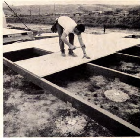
NAILING OF SUBFLOORING can be by hand or machine, using hardened screw-shank nails.
