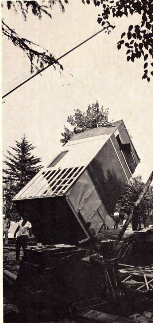
4. Third section, shipped on side, is tilted up.
