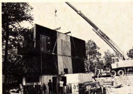
3. Second section is set on top of first.
