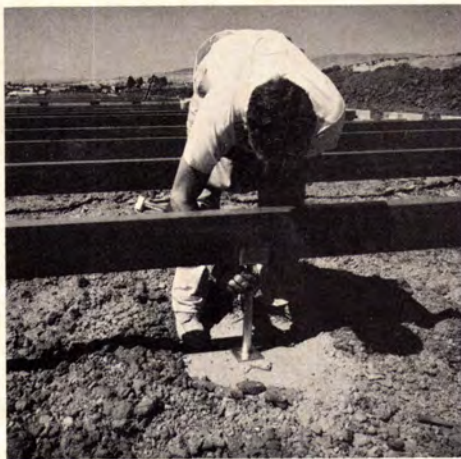
SCREW-TYPE JACKS are used to level beams, can be easily readjusted if foundation settles.
