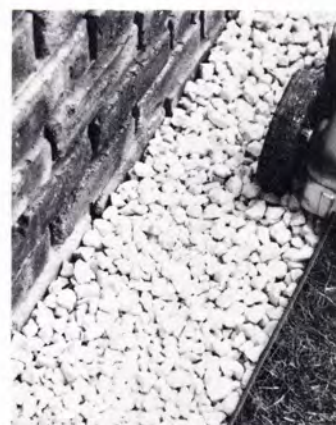
Landscape edging lets a mower ride over it. Interlocking steel strips, \frac{3}{16} " or \frac{1}{4} " thick, 4" or 5" wide and 16' or 20' long, have slots every 30" through which 16" steel stakes are driven. Black or green. Joseph T. Ryerson & Son, Chicago.
