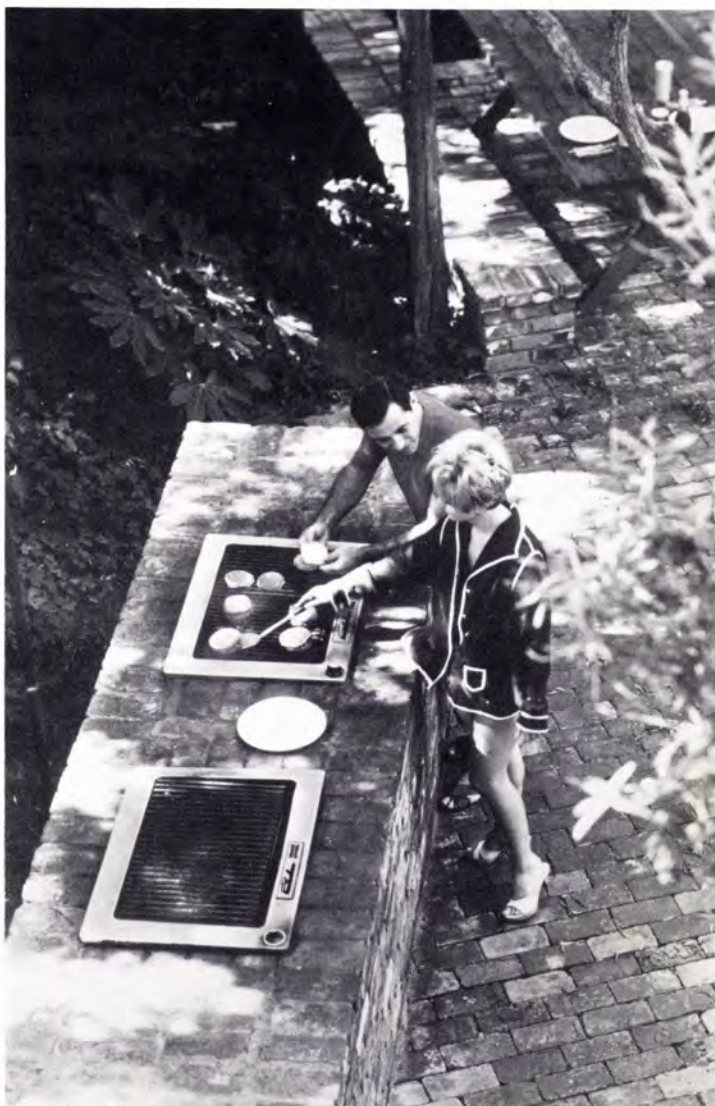
Gas-fired barbecues , shown built into an outdoor brick counter, have self-cleaning ceramic coals that never need replacing, provide intense, radiant heat for broiling ten minutes after ignition. Waste King Universal, Los Angeles. Circle 205 on Reader Service card
