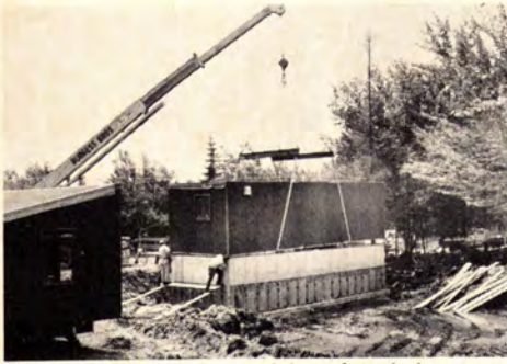
1. First section is lowered into foundation.
