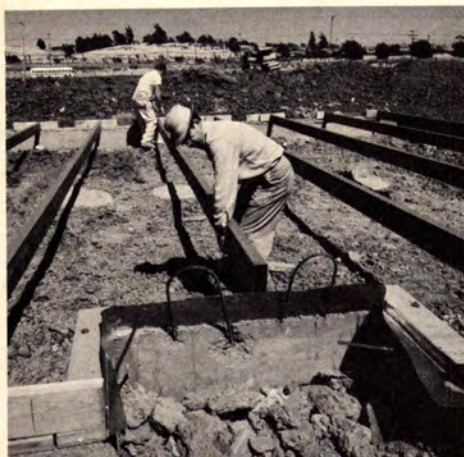
STEEL-BEAM PLACEMENT requires two men. Beams are delivered precut to specified sizes.
