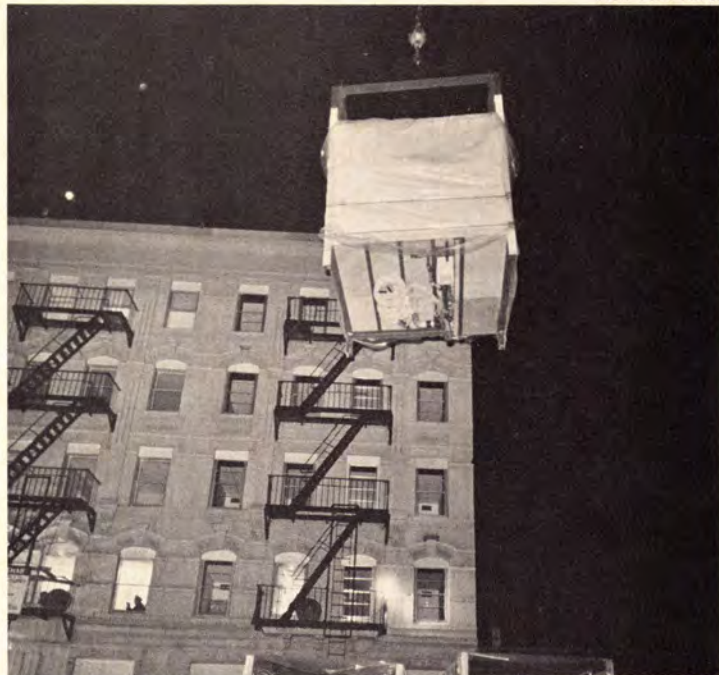
FLYING CORE full of costly equipment soars to place in highly publicized "systems" rehab project in New York City. Cost: $45 a sq. ft.
