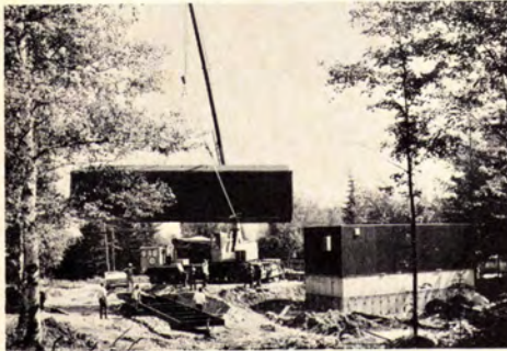
2. Second section is lifted from trailer.
