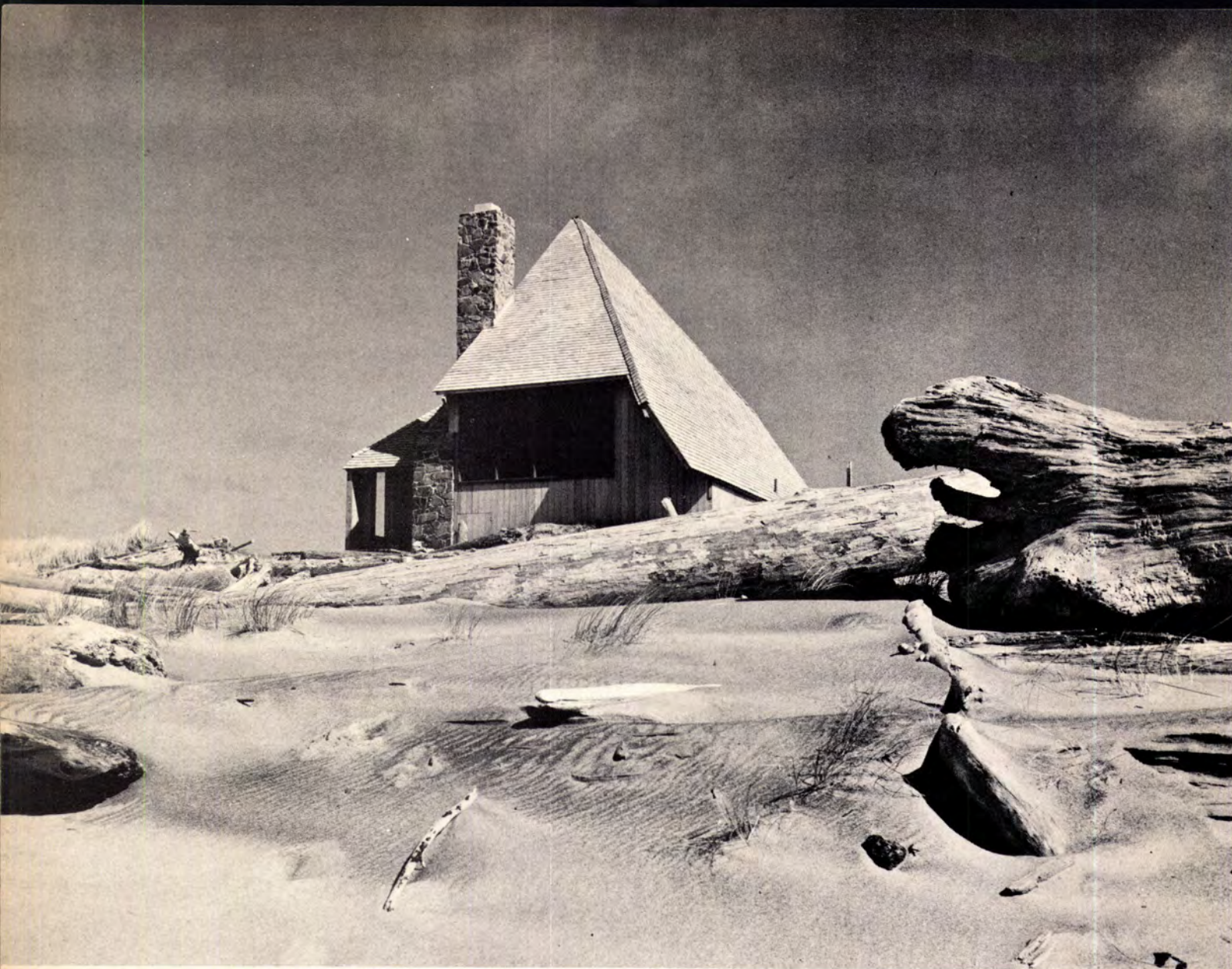
STEEP ROOF shelters large living room windows overlooking the ocean. Cedar shingles and siding will be left to weather naturally.
