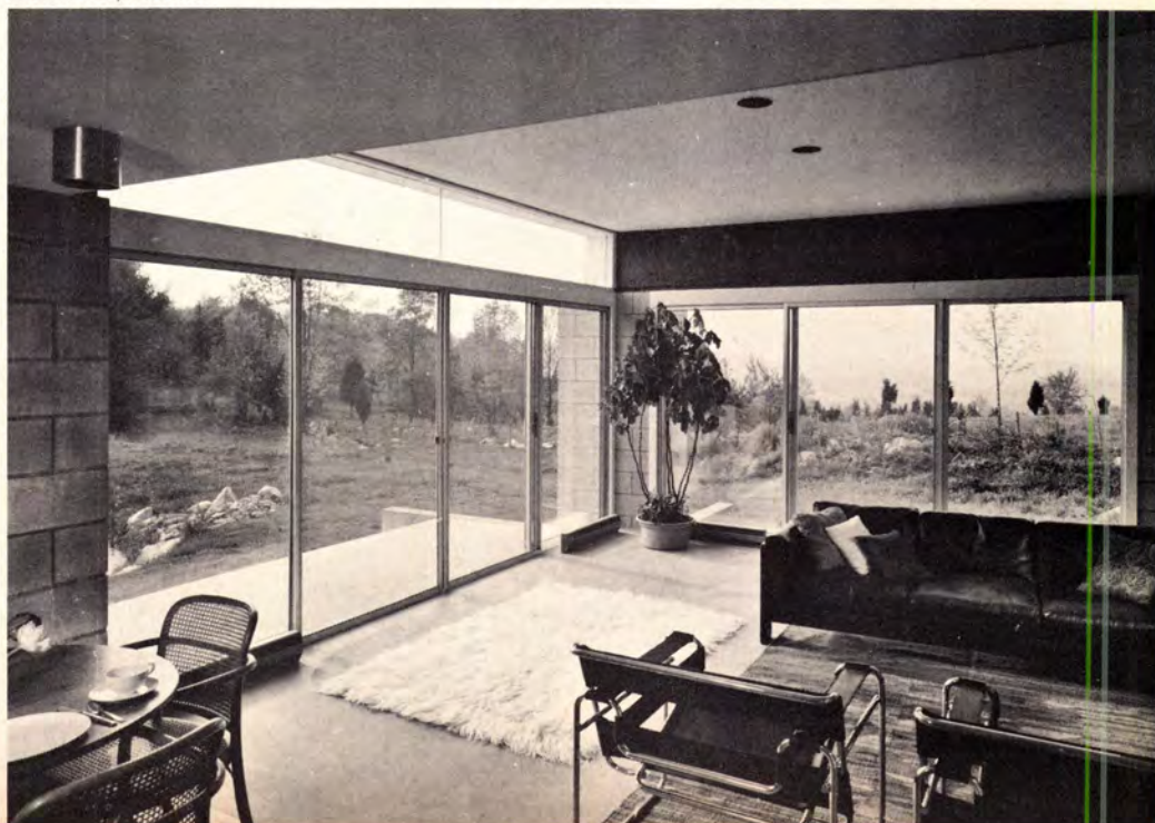
BEDROOM ( above ) and living room ( below ) are finished in concrete block on all outside walls. Both rooms have glass walls on two sides.
