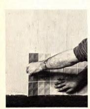
Pre-grouted tiles come in sheets of nine 41/4" x41/4" ceramic ceramic tiles that can be installed as one unit. Flexible grout permits the panels to be bent at the joints for corners or for curved surfaces. Grout strips fill between panel Amsterdam, New joints. Circle 310 on Reader Service card
