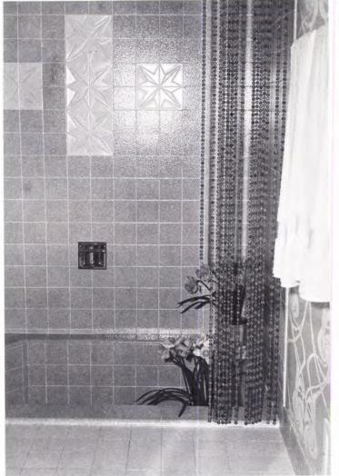
**Roman tub** is built into California production house, using ceramic tile. Decorative inserts and accessories are built into the wall, and each buyer is given a choice of color and pattern. Mosaic Tile Div., Stylon, Corona, Calif. Circle 325 on Reader Service card
