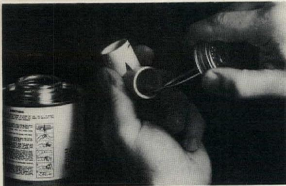
Remove surface gloss from the tubing end and fitting socket with CPVC cleaner or fine sandpaper and wipe clean with a dry cloth. Brush CPVC cement to the inside of the socket.
