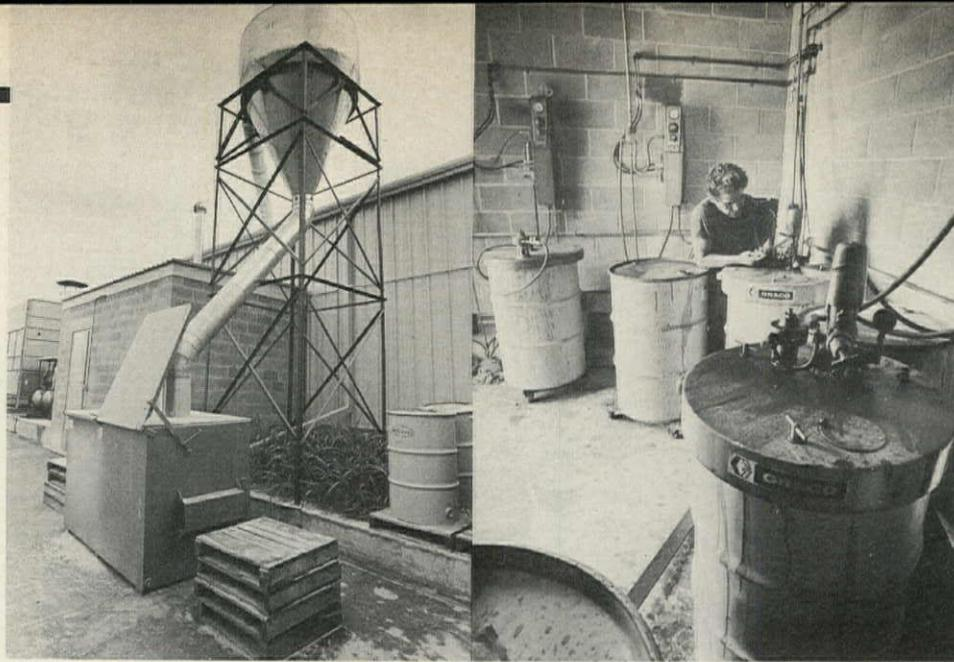
9 Air make-up system for spraying operation is shown in foreground of photo at left; behind it is shack from which paints (photo, right) are pumped into spray booths.
