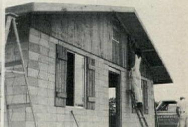
Low-cost block system needs no mortar. "Wedge Blocks" have twin V-grooves that interlock firmly so hollow cores align vertically. The house above is 25' x 28' with 8'-high walls, 992 ft. of interior walls, four doors, and seven windows. Masonry work was completed in two days at a cost of \$1,209.58. Blocks cost \$634.50; grout for the cores next to windows and doors and at corners cost \$18; and mortar
