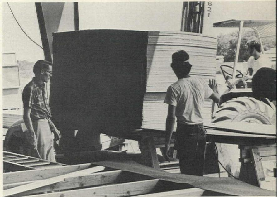
③ Load of sheathing is delivered by forklift to panel plant. From three to five weeks inventory of raw material is always kept on hand.
