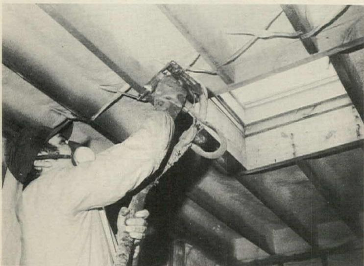
Low temperature foam system provides a good bond of the urethane foam to substrate or metal even at temperatures down to 28° F. Tested in Alaska's freezing weather, the foam adhered well, showed no
