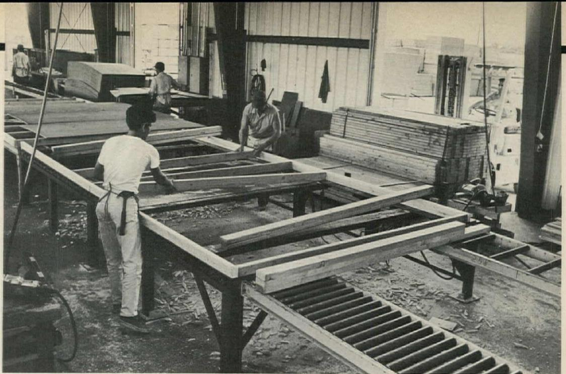
1 Studs are delivered through door at right, sheathing through door at upper left, right next to their points of use.
