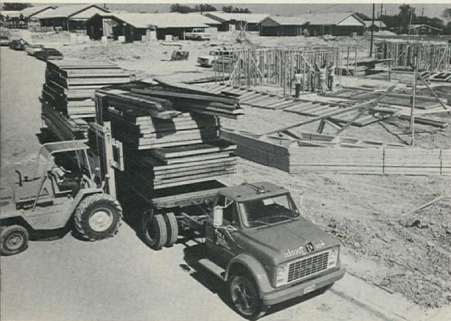
**6** Components are unloaded at site. Special ground-hugging float, 40' long (legal limit is 44'), carries two complete small houses.
