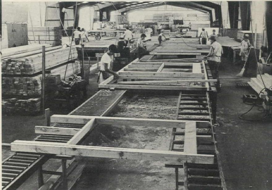
**3** Subcomponents—in this case, window frames—are made off the main panel assembly line, then installed in panels at this station.
