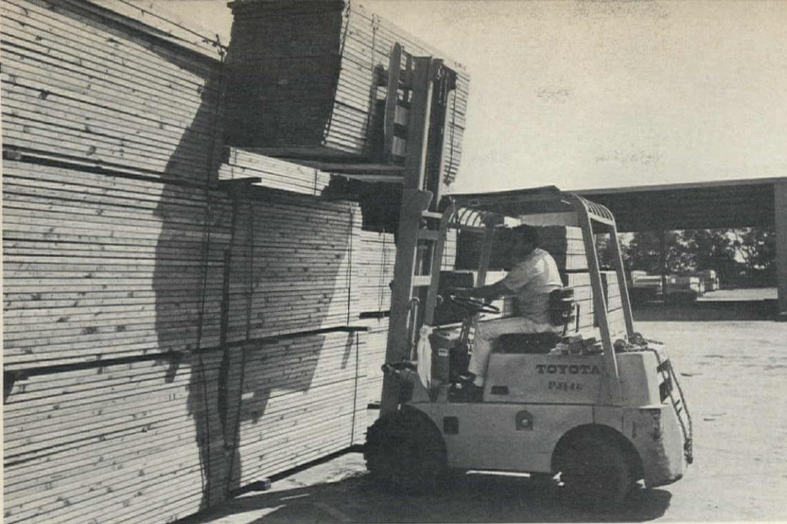
② Bundle of studs is put in raw material inventory in yard area. Building visible in background is panel fabrication plant.
