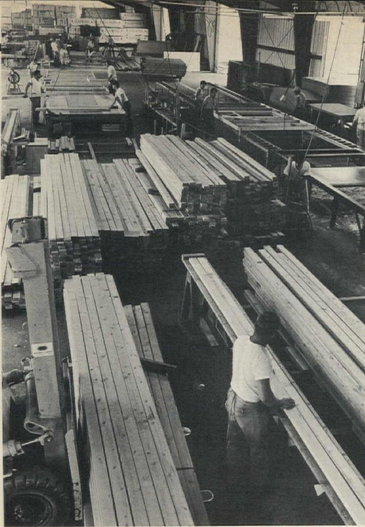
**2** Layout operation establishes lengths of panels, positions of openings, and special features. It stays half a day ahead of production line.
