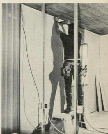
Pipe insulation is of rigid urethane. Shown being installed on dual temperature pipes in a 40-story apartment building in Boston, "Armalok" comes in easy-to-handle 4' lengths, speeds construction
