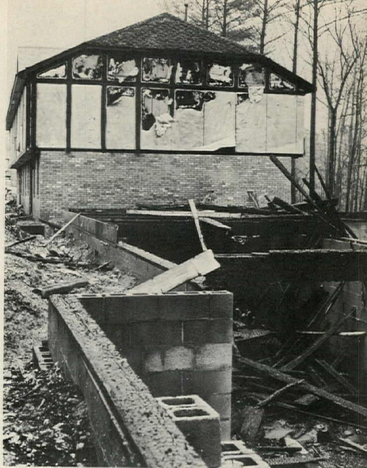
Fire retardant siding remains on the still-standing apartment building above. Fire started in burned-out buildings in foreground, was contained in them by the siding. "Panel 15" credited by fire de-
