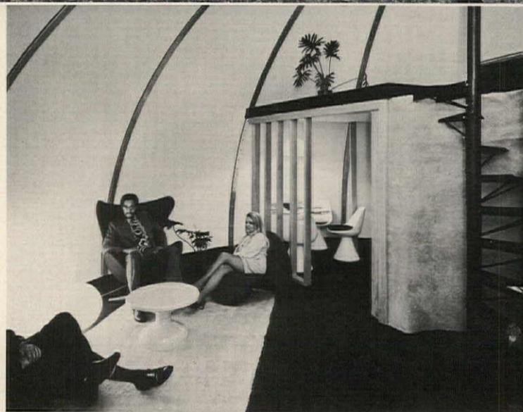
Interior view shows how the tapered panels are joined by aluminum ribs. Main living area is in foreground in front of kitchen-dining room. Spiral staircase leads to the loft.
