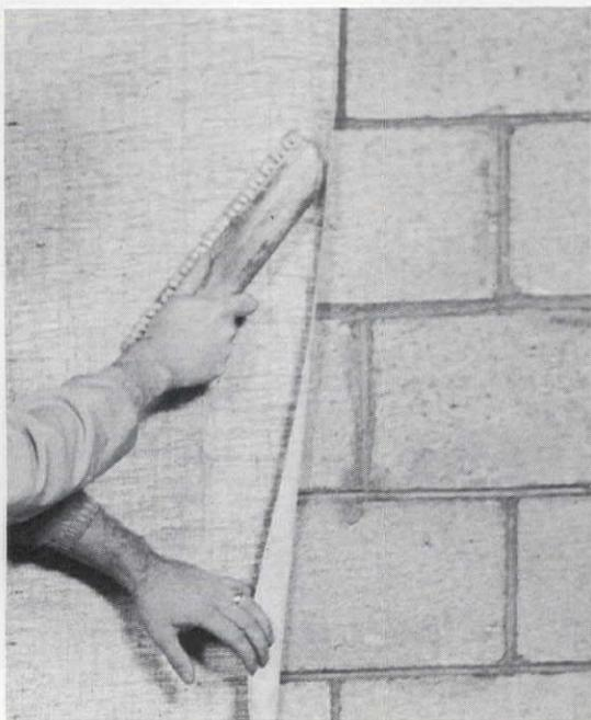
A fire-resistant roll of plaster in a scotch weave is used in the same way as conventional wallcoverings. Offered in 48"-wide rolls, the surfacing material can be directly applied with an adhesive to any rigid surface including concrete block. The covering remains flexible until it is applied at which time water in the adhesive sets the plaster. Flexi-Wall Systems, Liberty, S.C.
