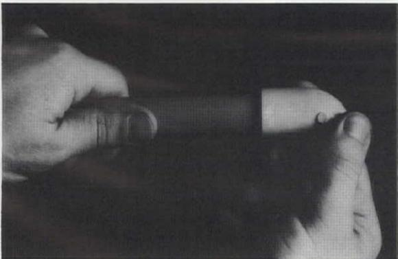
Push the tubing into the fitting. Then give either the tubing or the fitting a quarter turn to insure proper distribution of cement. Immediately adjust for direction. Wipe excess cement from the fitting lip; hold both together for a few seconds.
