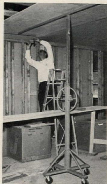
Wallboard lifting device has heavy-duty arms that lift and hold standard wallboard sections, up to 16' long, in position for seaming and nailing. Constructed of heavy steel tubing, unit has a gear drive assembly for raising and lifting and a hand wheel control. It is on wheels for easy handling. Astron, Findlay, Ohio.
