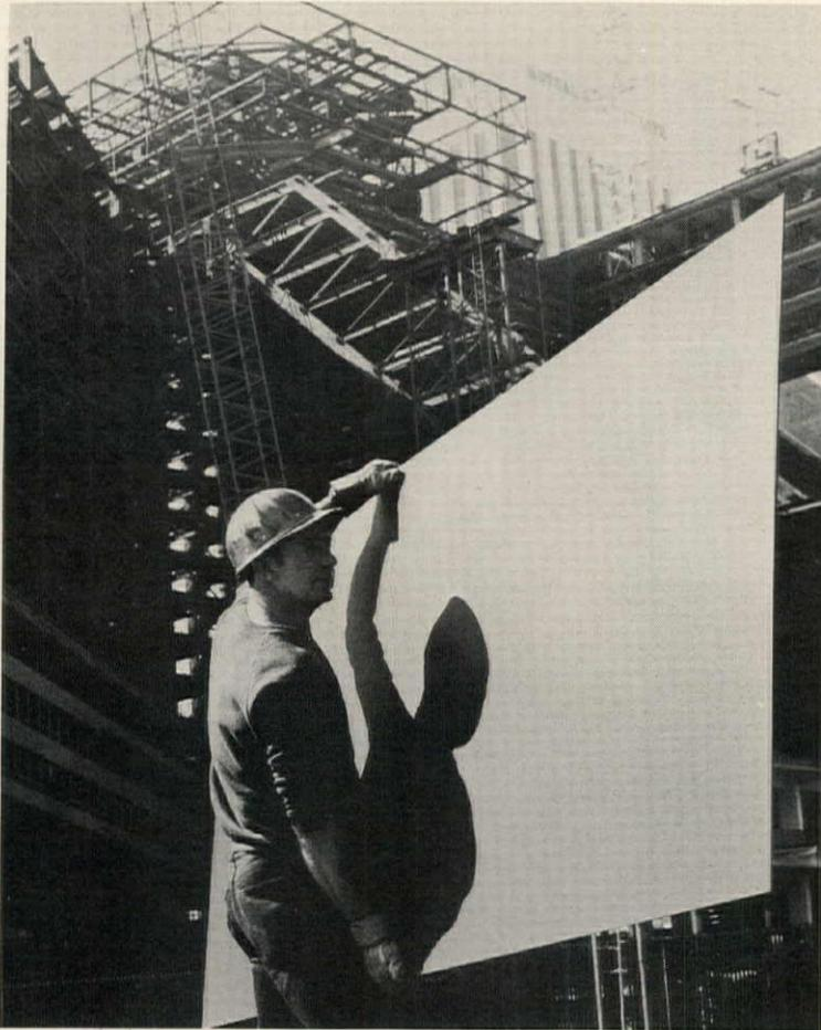
**Laminated building panels** are faced with integral color anodized aluminum. The lightfast anodic coating is resistant to corrosion and abrasion. Offered in medium or dark bronze, the aluminum comes as a
