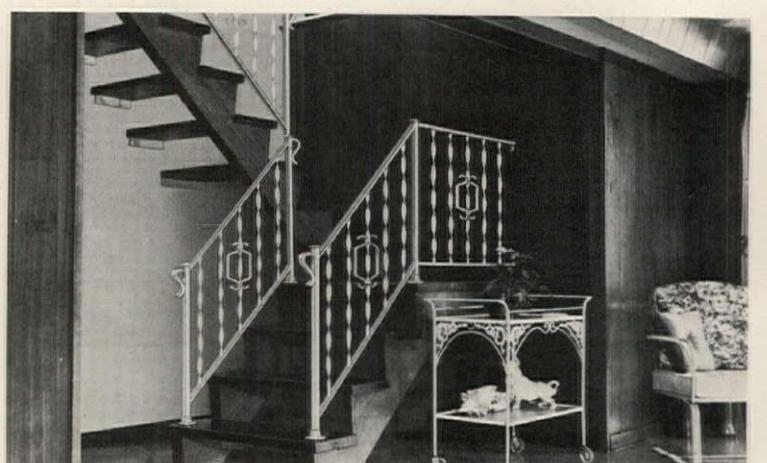
**Wrought iron railings** in 4', 5' and 6' sections can be pitched to fit any stair angle. The unitized, weld-free construction is suitable for interior or exterior installation. Parts are
