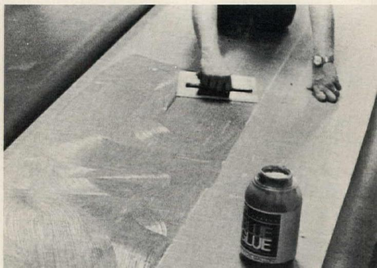
**Carpet adhesive** has coverage of 80 sq. yds. per gal., about 7 times the normal, which results in greatly reduced installation costs. Suitable for vinyl- and latex-backed carpet, the adhesive spreads thin and even. 3M, St. Paul, Minn. CIRCLE 237 ON READER SERVICE CARD
