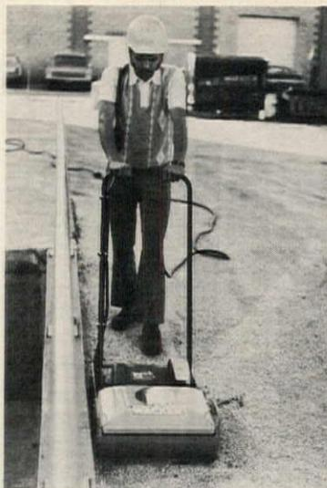
Electrically driven vibro plates that compact granular soil as well as hot and cold asphalt mixes control air and noise pollution. Exhaust emission and accompanying noise common to similar tools with gasoline engines are eliminated. Shown are
