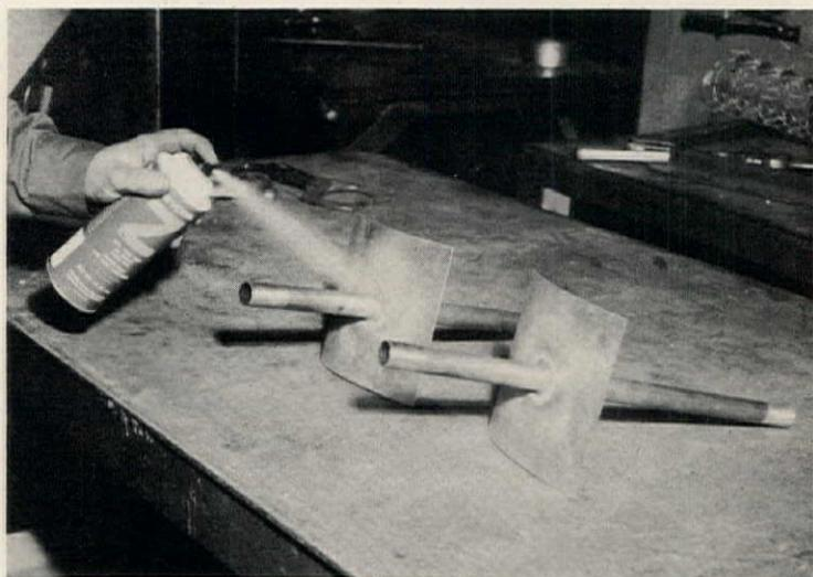
**Galvanizing compound** in an aerosol can may be applied to any iron or steel surface. The crack-resistant, rustproof coating, containing 95% zinc, eliminates hot-dip galvanizing. It can be used alone or under paint. Devcon, Danvers, Mass. CIRCLE 240 ON READER SERVICE CARD
