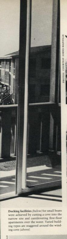
Entrance elevations are curtain-walls fabricated of timbers and low-maintenance asbestos-cement panels with factory-applied, long-life finish (Permatone).
