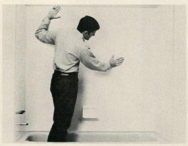
Fiber glass tub surround is easily installed over any hard, solid surface. No grouting, mitering or edge moldings are required. Side pieces wrap around to form part of the CIRCLE 202 ON READER SERVICE CARD
