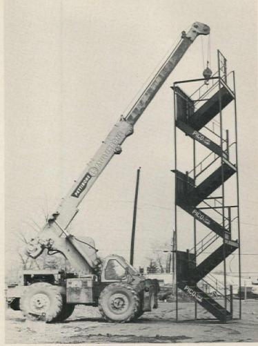
Prefabricated, pre-erected stairs are suitable for use in masonry, concrete, steel or wood structures and precast systems. Each steel tower contains a complete staircase up to 40' high including treads, risers,
