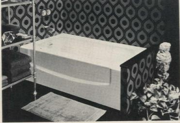
Acrylic-faced fiber glass bath unit, designed to meet the needs of small-volume contractors, is 30 lbs. lighter than a comparable steel tub. "ACRA-BATH" combines the strength and lightness of a fiber
