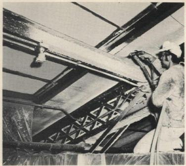
Spray-on fireproofing for exposed structural steel beams and columns provides protection for up to four hours. Fire heat causes a chemical reaction in "Pyrocrete" during which cooling water vapor is released. This cooling agent protects the steel against structural failure. Carboline, St. Louis, Mo.
