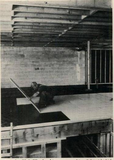
Non-combustible building board is made of 100% recycled wood fiber material that has been impregnated with chemicals to protect against flame-spread, termites, rot, fungus and moisture. The substance is compressed into lightweight highdensity, insulation boards in <sup>15</sup>/<sub>32</sub>" or 5%" thicknesses and sizes of 4'x8', 4'x12', 8'x8' and 8'x12'. Homasote, West Trenton, N.J. CIRCLE 214 ON READER SERVICE CARD
