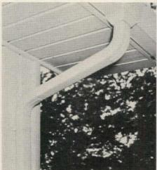
Soffit panels that resist warping. They're strong but light, easy to handle and cut.
