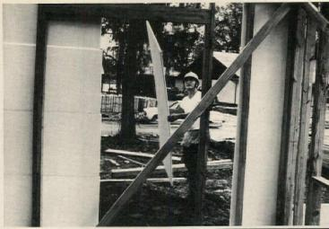
Rigid plastic foam insulation functions as nonstructural sidewall as well and requires no vapor barrier. T&G edging runs on all four sides of the lightweight boards providing leakproof mating. On-site tailoring of window and door areas is easily accomplished by cutting material with a sharp knife. AMSPEC, Columbus, Ohio
