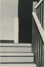
Yellow safety strips of polyvinyl chloride signal a warning. They eliminate the need for constant painting and maintenance. Available are stair nosing marker for concrete stairs, pipe rail marker for railings or gate applications and corner guards for edges of equipment. Pawling Rubber, Pawling, N.Y.
