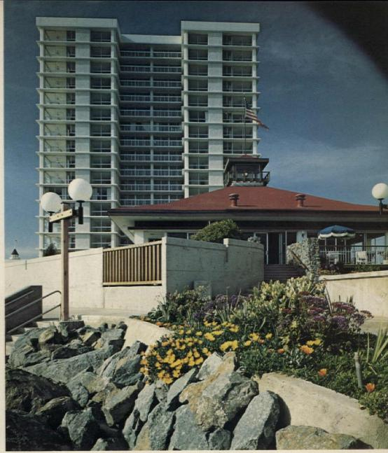
Stone seawall (above), a \$500,000-construction job, forms and shapes the beach, which was showing signs of erosion. Some 10,000 stones, weighing up to ten tons, were brought in from a nearby quarry.
