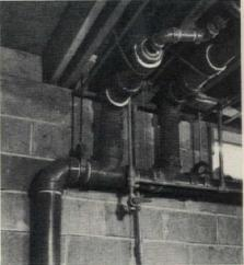
CPVC water supply pipe and PVC DWV resist build-up of hard water deposits and reduce heat loss
