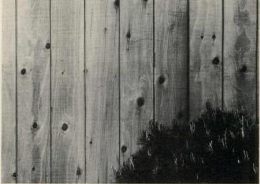
Redwood plywood siding panels bleaching. Standard 3/8"- and 5/8"rugged finish provides for natural Portland, Ore. weathering, staining, painting or
