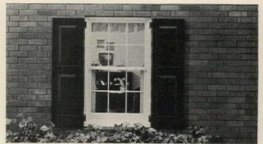
Vinyl shutters are hung on predrilled black brackets that simulate hinges to provide an authentic look. Available in panel or louver styles, shutters are of high-impact vacuum-
