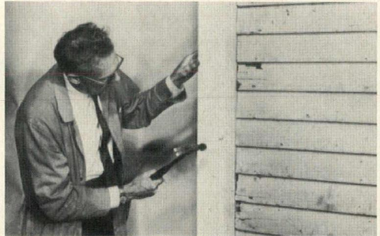
**2. Corner posts.** Place posts on all inside and outside corners, allowing  $\frac{1}{4}$ " at the top. Position the post by placing nail at top of upper slot, placing all other nails in the center of the slots.
