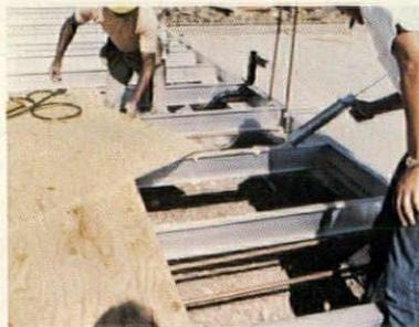
Alumiframe members are strong. They're made of the same architectural alloy used to make bridge railings and overhead highway sign trusses. And because they're extruded, each member has the metal distributed exactly where it's needed for maximum strength and function.
