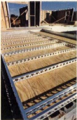
Because Alumiframe members nest together, they require a minimum of storage space. Aluminum's light weight simplifies materials handling. Jigs can be quickly rigged to produce multiple panels. Radial arm saws trim Alumiframe plates
