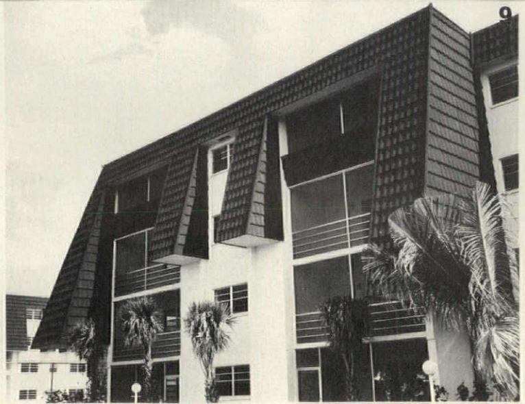
**Terne-coated stainless steel (TCS) (1)** is used on the salt box roof and canopy shown. TCS accepts paint without the need for undercoating or can be allowed to weather naturally. The versatile metal is resistant to salt air and weathering. Follansbee Steel, Follansbee, W. Va.
