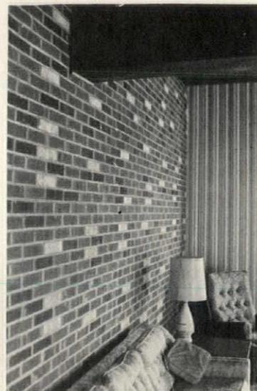
Easy-to-install thin bricks for interior application are the same height and width as traditional bricks but are only 1/2" thick. Brick wall is applied by spreading a layer of mastic on the surface to be covered and pressing the Brickettes® into place. Available in 12 color blends. Modern Methods, Evansville, Ind.
