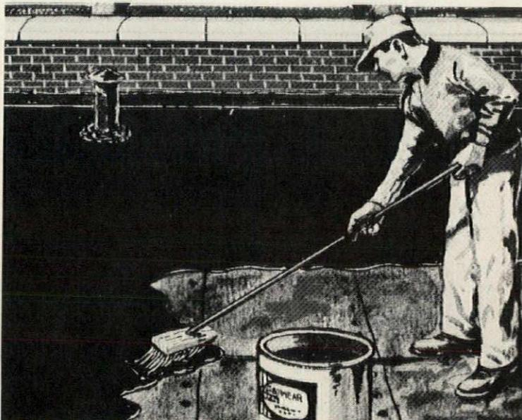
Roofcoating is suitable for repair applications in all types of weather. Thick, heavy, cold-process "Barrow-kote" is a plastic-type product that can be applied by brush or spray. The roofcoat penetrates only enough to lock into the old roof base without disturbing the composition to which it is applied. Consolidated Paint, Cleveland, Ohio. CIRCLE 246 ON READER SERVICE CARD
