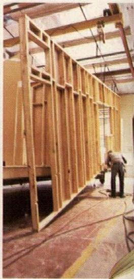
So it was a simple and logical step for Levitt to expand its California mobile home business into the sectionalized housing market. The same production line produces a mix of mobile and sectionalized homes at the rate of five "floors" per day.
