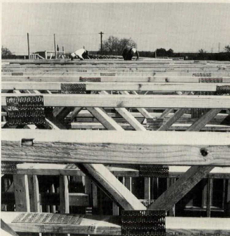
Floor truss system saves on-site labor. Trusses feature an open web construction that permits installation of duct-work, heating, electrical wiring and plumbing without additional carpentry. Narrow 2'x4' trusses eliminate large floor members that can limit building design. Easy-to-install units need no steel hangers and bridging. Evans Products, Portland, Ore.
