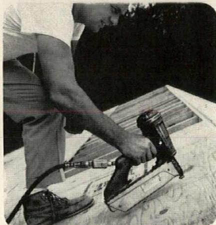
Staple Nailer anchors down plywood roof deck
