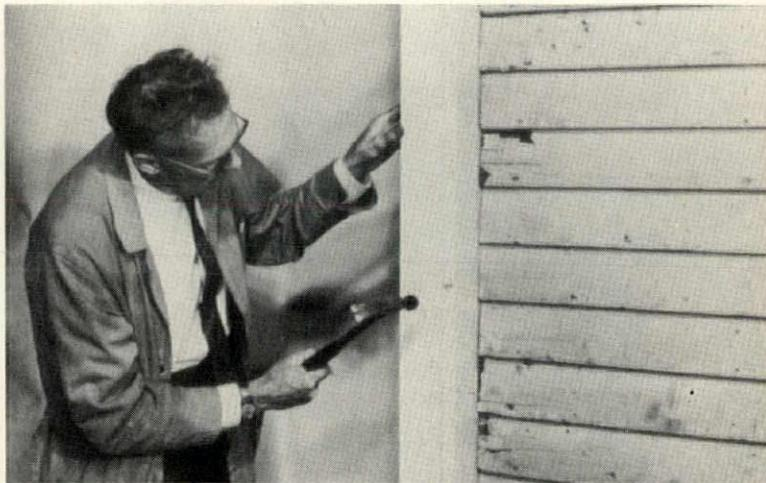
**2. Corner posts.** Place posts on all inside and outside corners, allowing  $\frac{1}{4}$ " at the top. Position the post by placing nail at top of upper slot, placing all other nails in the center of the slots.
