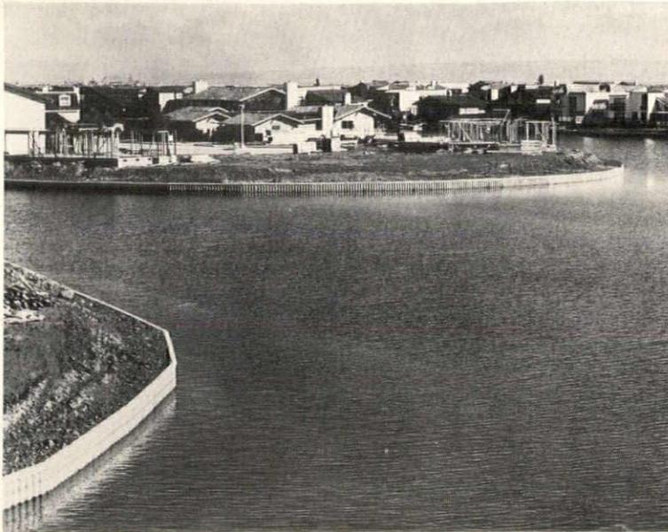
**Marine retaining-wall system, Shore All™** protects waterfront property from the sea. A special corrosion-resistant corrugated bulkhead is formed from sheets of durable aluminum. Sheets are joined by sand-tight ball-and-socket joints and capped with an aluminum alloy extrusion that is bolted into predrilled holes. Kaiser, Oakland, Calif. CIRCLE 231 ON READER SERVICE CARD
