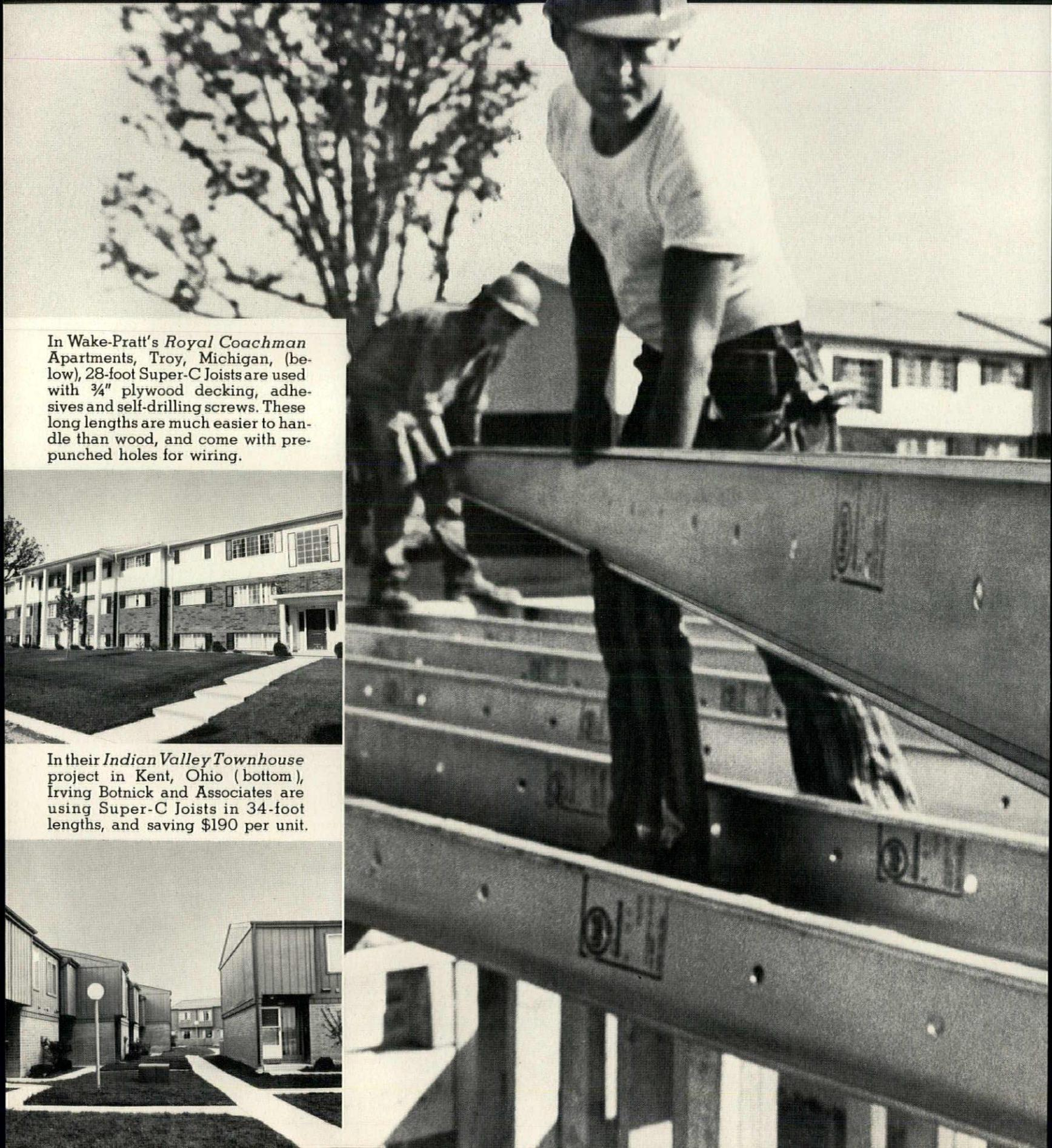
In Wake-Pratt's *Royal Coachman Apartments*, Troy, Michigan, (below), 28-foot Super-C Joists are used with  $\frac{3}{4}$ " plywood decking, adhesives and self-drilling screws. These long lengths are much easier to handle than wood, and come with pre-punched holes for wiring.
