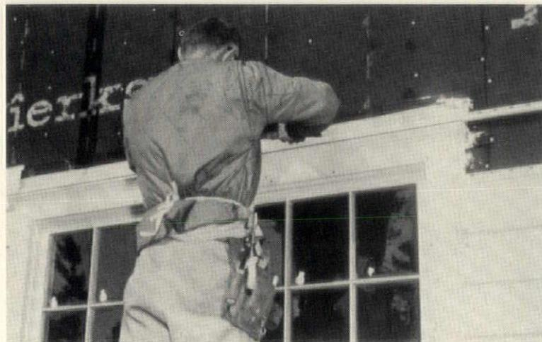
**8. Fitting around window.** Nail J channels on window and door sides and tops, and undersill trim on window bottoms, to receive siding. (Vinyl window head flashing should be used above doors and windows unless previously flashed.)
