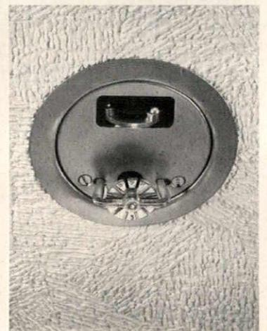
Recessed sprinkler, "Aquamatic," provides fire protection and blends with room decor. Each sprinkler, controlled by heat sensitive bimetallic discs, operates independently. Units will shut themselves off after extinguishing a fire and turn themselves back on if the fire rekindles. Grinnell, Providence, R.I. CIRCLE 205 ON READER SERVICE CARD
