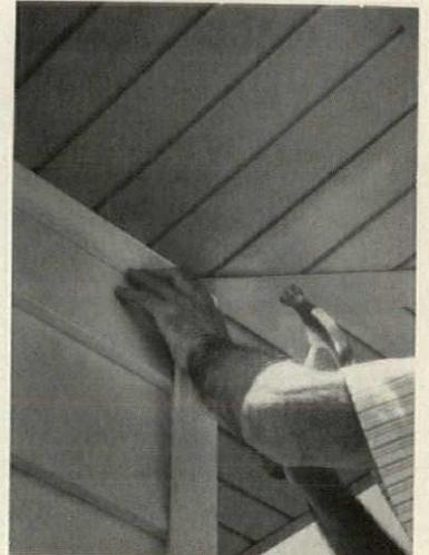
**Aluminum soffit and fascia system** is available in a choice of white, yellow, brown, green or gold, to match any styling. Prefinished panels, matching fascia and trim, combine the rich appearance of select grade wood with the low-maintenance characteristics of aluminum. Material will not rot, split or rust. Kaiser Aluminum, Oakland, Cal.
