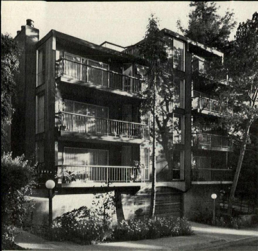
Concrete and masonry garage (above), tucked under the rear of the three-story and penthouse frame building, was designed to conform to the slope of the 38,650 sq. ft. site. Rooftop laundry facilities (not visible) serve all tenants.
