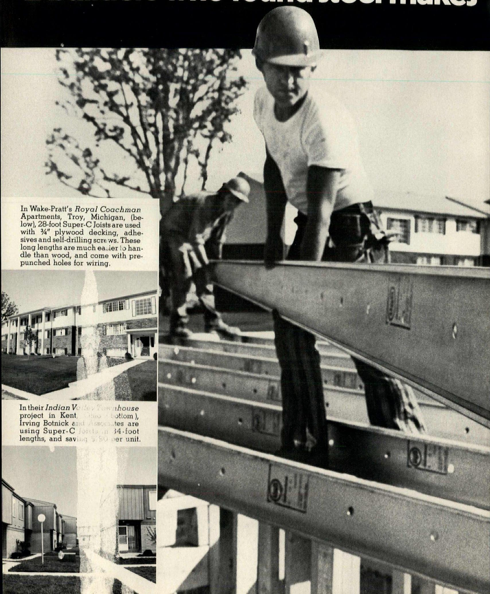
In Wake-Pratt's *Royal Coachman* Apartments, Troy, Michigan, (below), 28-foot Super-C Joists are used with  $\frac{3}{4}$ " plywood decking, adhesives and self-drilling screws. These long lengths are much easier to handle than wood, and come with pre-punched holes for wiring.
