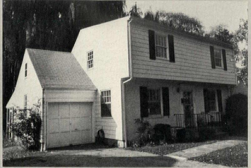
**\$5,000:** Removed half of old roof and installed shed dormer with two windows; owner installed interior partitions, insulation and drywall.
