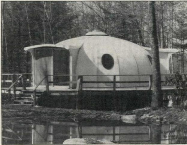
Dealerships are now available for O'Dome, the exciting and successful year round vacation home that sells for the price of a car. The O'Dome has 510 square feet of living space and features tough, durable fiberglass and urethane foam construction, providing excellent insulation and maintenance-free living. Low-cost shipping anywhere. Prospective dealers must be able to demonstrate an
