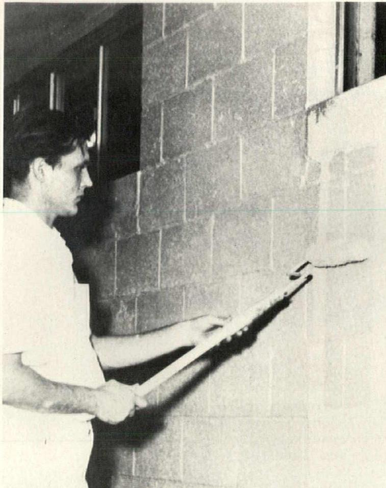
**Water-based epoxy resin, "Dur-A-Poxy,"** works well on moist or wet surfaces. Easily applied with a brush, spray or roller, the coating is odorless, fire resistant and has a low toxicity. Suitable for use on concrete, cinder-block or wood, the material is resistant to solvents, acids and alkalis. Dur-a-Flex, Hartford, Conn. CIRCLE 225 ON READER SERVICE CARD
