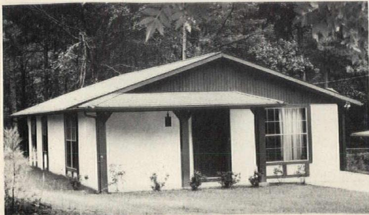
**Simple structural system**, shown in a completed house, consists of building blocks and a mortarless surface bonding cement, Surewall®. The blocks are stacked in a running pattern; then the bonding cement is mixed and troweled onto the sides providing a smooth, white, moisture resistant finish. W. C. Bonsal, Lilesville, N.C. CIRCLE 212 ON READER SERVICE CARD
