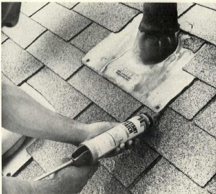
**Instant Patch® roof repair** contains both organic and inorganic fibers. It dries to a tough, long-lasting membrane that stops leaks and rebuilds worn-out roofs and flashings. Available in convenient 11-oz. cartridges or in quart, gallon or 5-gallon cans, the material won't shrink, sag, or run. Tremco Mfg., Cleveland, Ohio. CIRCLE 226 ON READER SERVICE CARD
