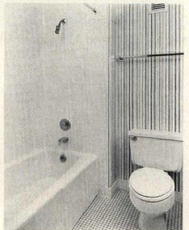
Finished bath is part of utility core. American Olean, Lansdale, Pa., supplies "Redi-set" adhesive-backed tile sheets drilled to production specifications.
