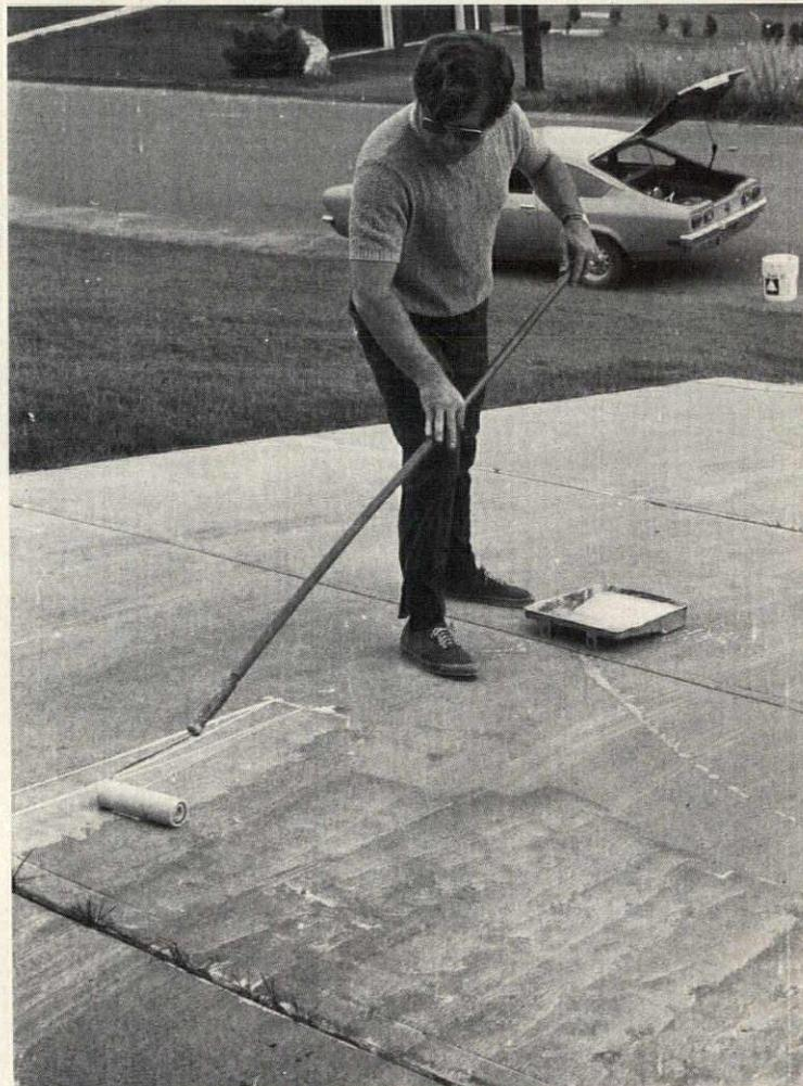
Non-flammable coating for concrete surfaces, "Sidewalk Saver," prevents cracking, chipping and spalling. The non-toxic, non-corrosive substance is suitable for use on steps and driveways as well as sidewalks. Easy to apply with a roller as shown, the coating cannot harm trees, shrubs or grass. International Salt, Clarks Summit, Pa. CIRCLE 267 ON READER SERVICE CARD
