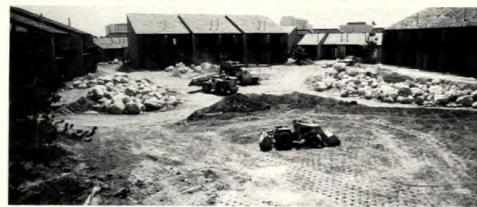
2. Soil cement is mixed into the lake bed and a sheepsfoot roller is used for compaction. Then locat of water-circulation piping—to be buried 18" to 24" deep—are outlined with lime
