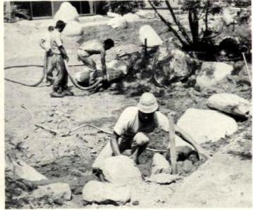
8. Earth-colored concrete is pumped between boulders along shoreline to hold them in place and to keep the shoreline from eroding.
