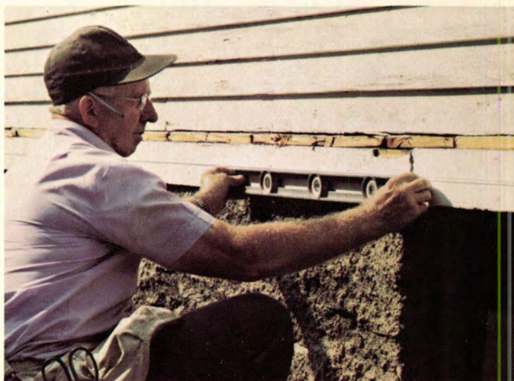
1. Check to see that all sidewalls and base are level and plumb. Snap chalk line for the starter strip.
