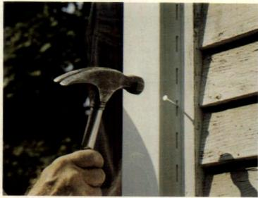
2. Install all inside and outside corner posts. Leave 1/4" at top. Finish nailing every 10" to 12" in the center of the slots.
