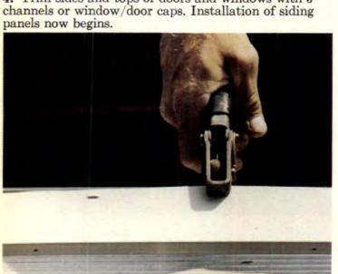
8. To fit a panel under a window, cut undersill trim the width of the opening and nail in place. Crimp the under window portion of panel with snap lock punch.
