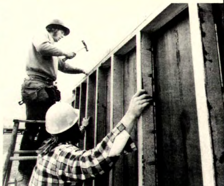
Composite 2x4, "COM-PLY," consists of a core of 1 1/2"x2 3/8" strips of particle board with 1/16" high-strength solid wood veneer laminated to each narrow side. Straight, durable studs are easy to nail. Georgia-Pacific, Portland, Ore. CIRCLE 256 ON READER SERVICE CARD
