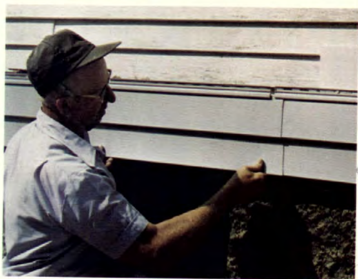
5. Snap bottom panels into the starter strip and nail. Backer board can be used for extra insulation.
