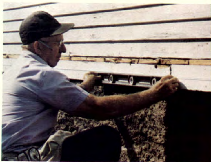
1. Check to see that all sidewalls and base are level and plumb. Snap chalk line for the starter strip.
