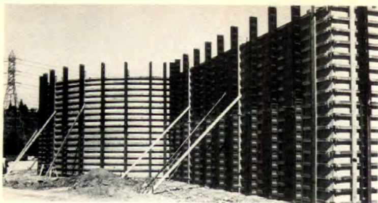
Concrete forming system, "Major Slim Soldier," is for fast, high pours that impose high form pressures. Cold-rolled steel vertical members have continuous corrugated web plates. Burke, San Mateo, Calif. CIRCLE 248 ON READER SERVICE CARD
