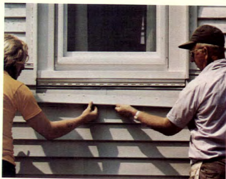
9. Slide the panel into the undersill trim. Installation of the top course follows a similar procedure.
