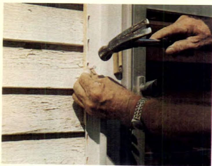
4. Trim sides and tops of doors and windows with J channels or window/door caps. Installation of siding panels now begins.
