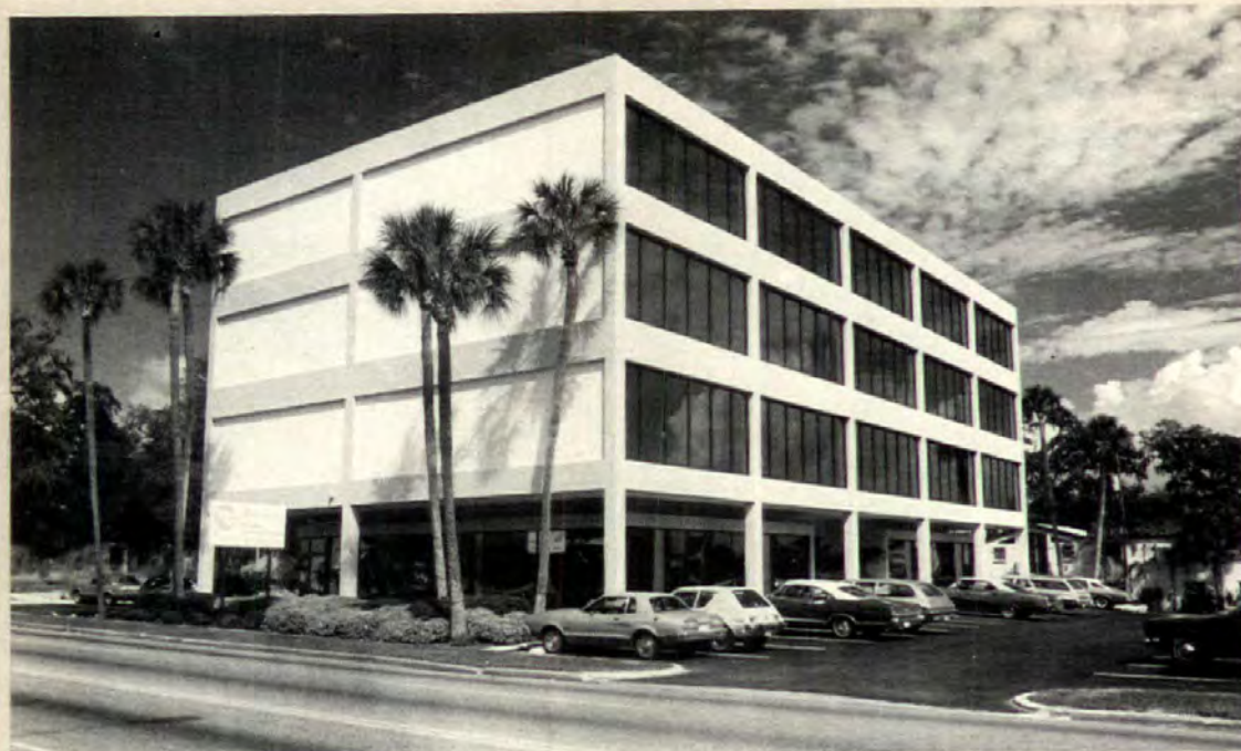
Exterior improvements of four-story office building (above) included a new finish—sand-toned acrylic—and solar control with reflective window film. Formerly open lobby was enclosed with glass walls and doors, carpeted and decorated with supergraphic (right). Trees, shrubs and white pebble ground cover dressed up lobby entrance (below).
