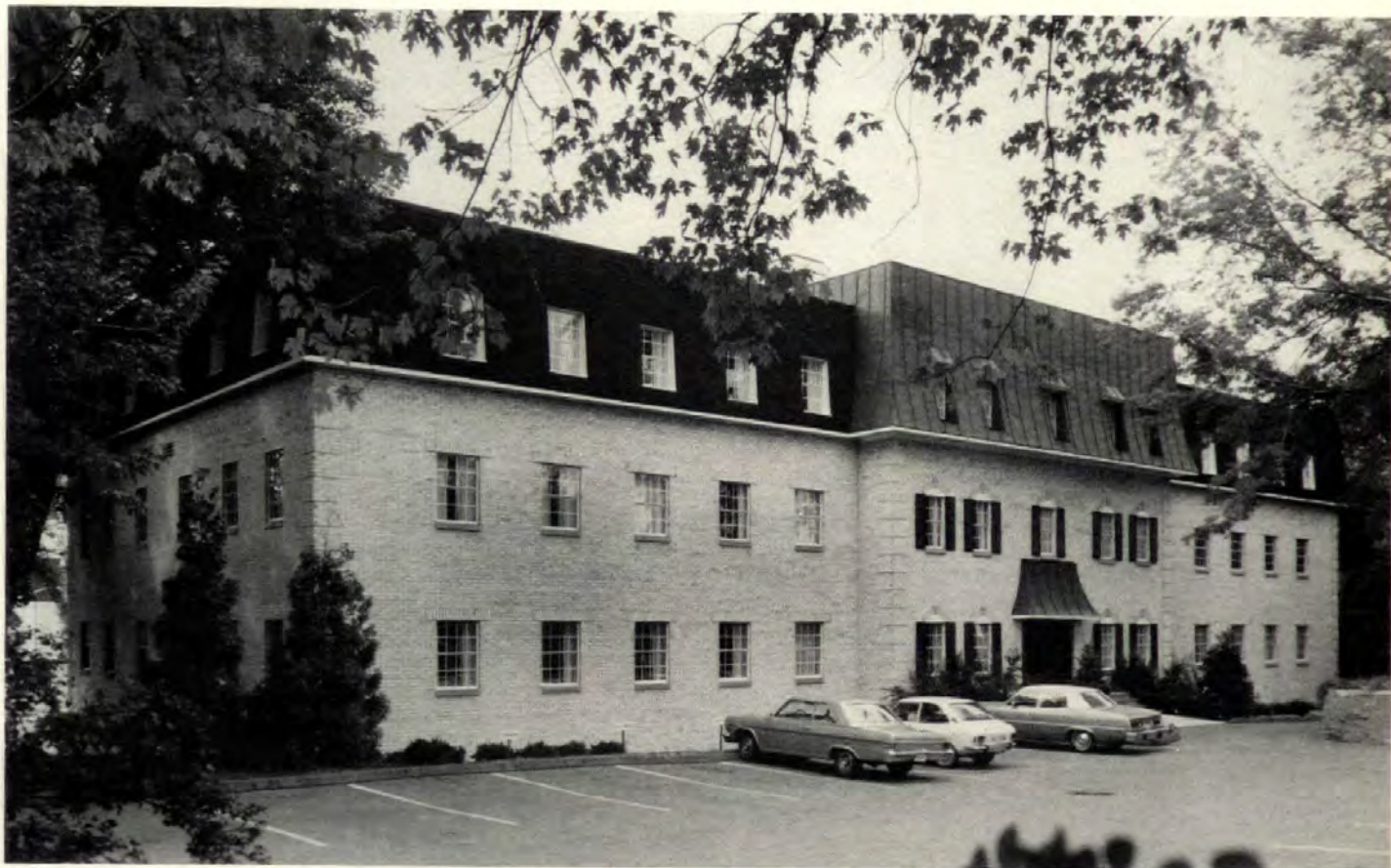
Mansard-roof facing and rearward sloping terrain make this new office condominium appear lower than its actual four stories.
