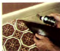
Tredway installs over concrete with just a band of adhesive.
