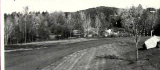
Narrowed natural-drainage street (above) eliminates need for most sidewalk, parking lanes and curbs used conventionally (below).
