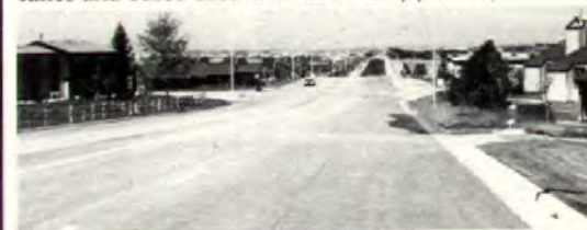
Narrowed natural-drainage street (above) eliminates need for most sidewalk, parking lanes and curbs used conventionally (below).
