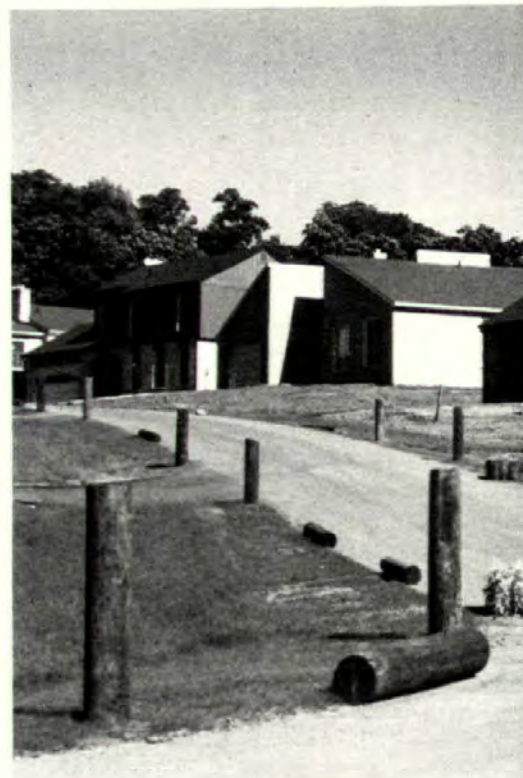
Bollards substituted for curbs in photo above keep traffic from running up on property and mark pavement limits for snowplowing.
