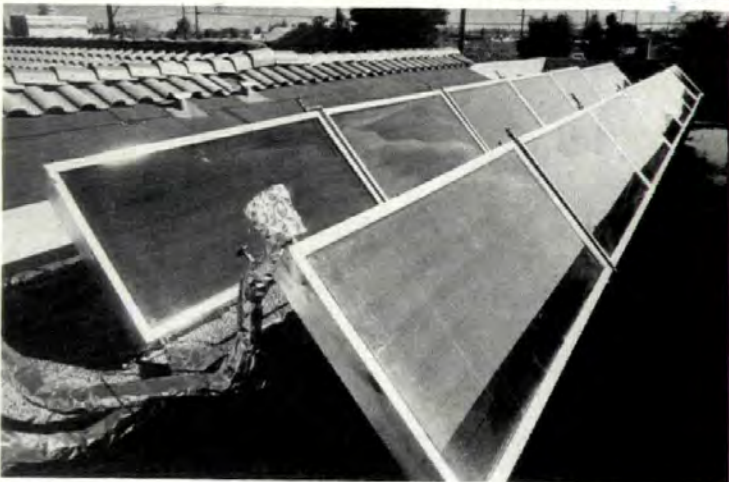
Solar collectors , angled at 45° (photo above) are installed on flat portions of roof. The collectors are masked by a parapet so they cannot be seen from the street (photo top of page).
