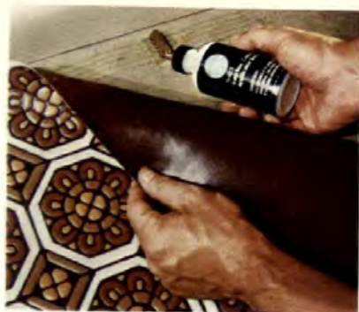
Tredway installs over concrete with a band of adhesive.
