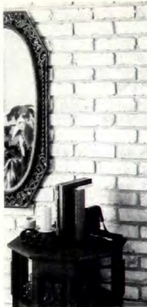
Simulated brick panels (above) are easy to install with nails or adhesive. Lightweight 6- or 12-brick panels come in shades of brown, beige and rust. Marlite, Dover, OH. Circle 223 on reader service card
