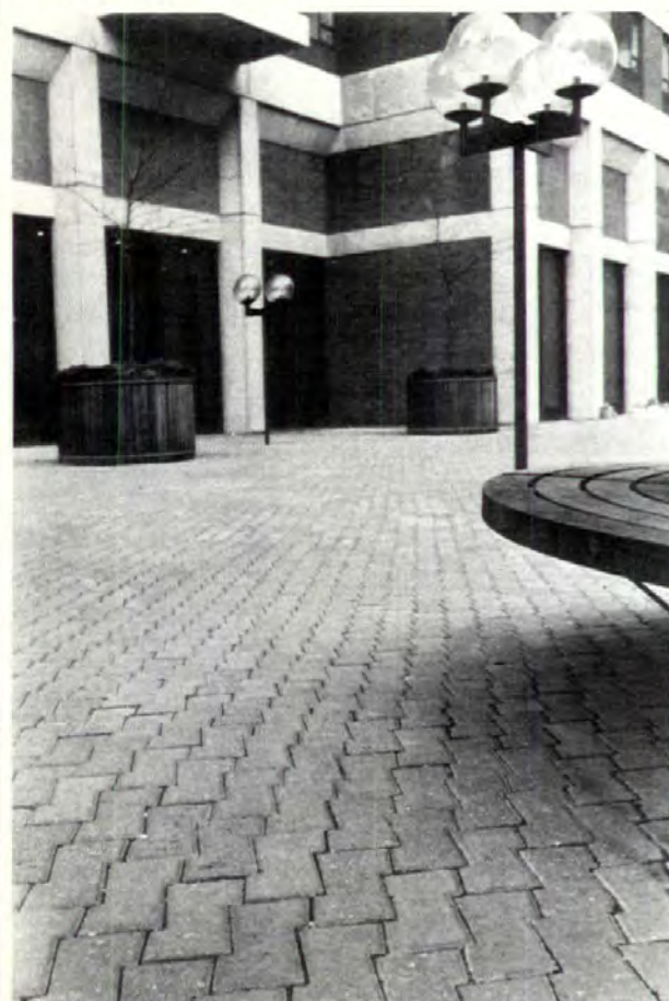
"Z" pavers (above) can withstand heavy traffic and severe weather conditions. Interlocking units, composed of clean-washed aggregates and cement combined in a "no-slump" concrete mix, are not slippery. Art Cement, Wilbraham, MA. Circle 244 on reader service card
