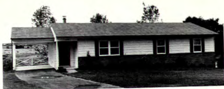
NAHB energy saver, clad in brick and aluminum siding, is similar in appearance to other houses constructed by builder David Smith. A typical wall section is shown below.
