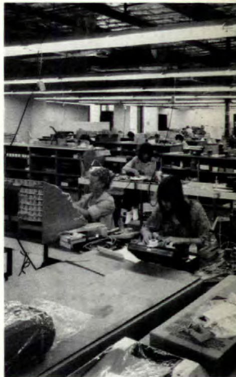
Component assembly area (above) occupies about 60% of the building. Note the absence of interior partitions, which allowed the space to be designed as one open area.
