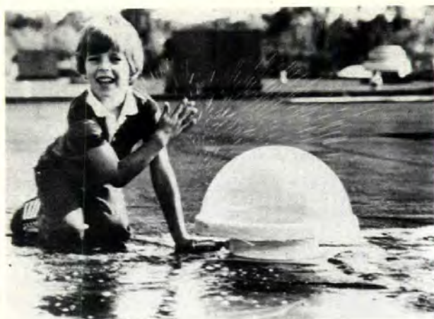
Solar-powered drain (above) provides low-cost, low-maintenance roof drainage. The compact 20-lb. unit pumps up to 1/2 gal. of water per minute from the roof. B. F. Goodrich, Akron, OH. Circle 211 on reader service card
