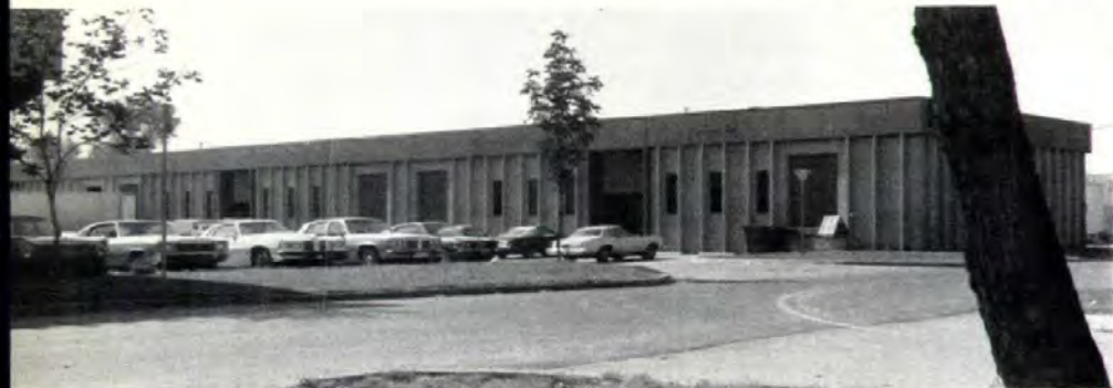
Small-user warehouse, built of precast concrete, is column-free inside so that space can be divided to specific tenant requirements. Architect: Herman Scharhag.
