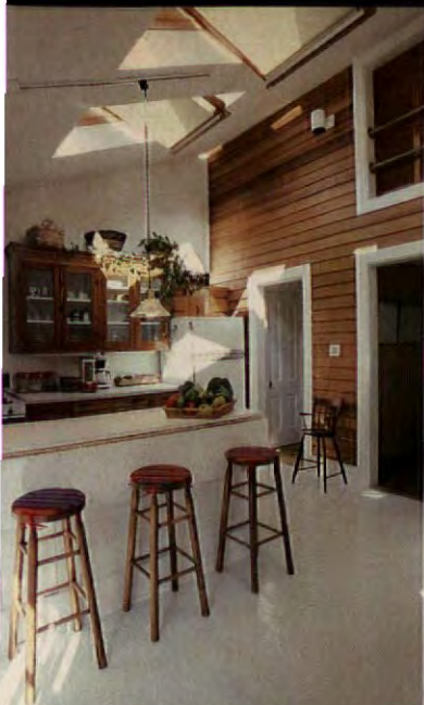
Double-glazed skylights warm the kitchen. Cedar boards mark the original outside wall.
