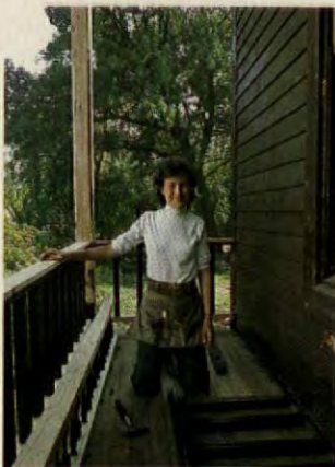
Salvaged materials and on-the-job carpentry skills yielded Emily a new porch.
