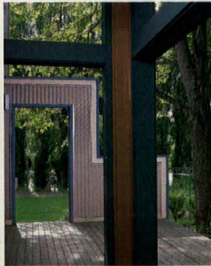
Panels of enameled corrugated steel (above and opposite) sheathe the Seattle house.
