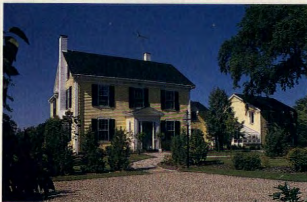
A connecting passageway satisfies the homeowners' requests for a new side entrance, a large greenhouse, and a shelter for their dogs in cold New England weather.
