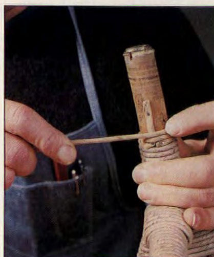
3. For unraveled wrap, first cut off and tack down end of old wicker. Tuck and tack new wicker end; wind tightly.
