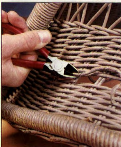
5. To reweave, first snip out broken or damaged wicker material (from underside) where spokes will support cut ends.
