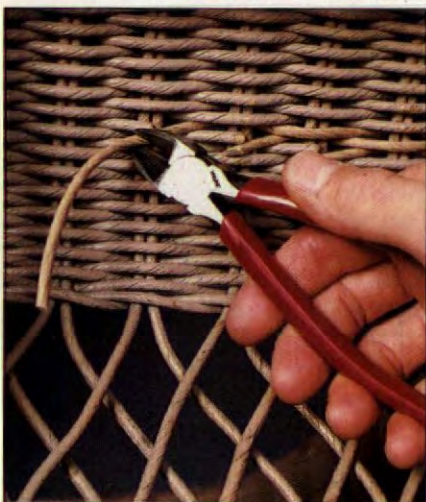
7. Snip off the ends of the new wicker repair from below, where the cut ends will "lock" against the supporting spokes.
