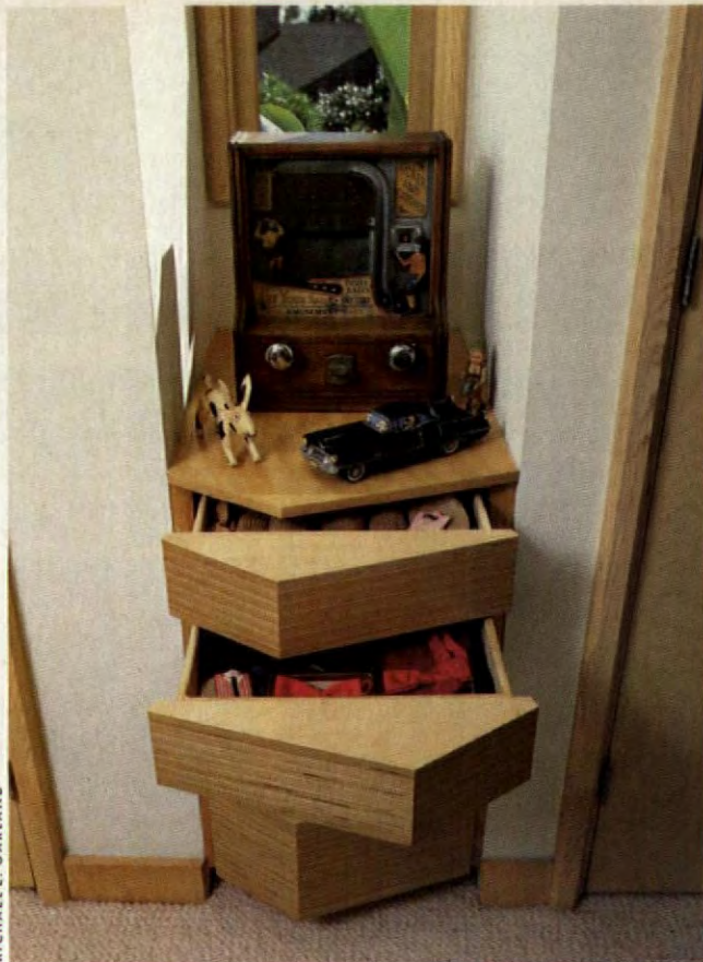
Laminations of Baltic birch plywood were used to sculpt the unusual drawer-front geometry of this built-in dresser.
