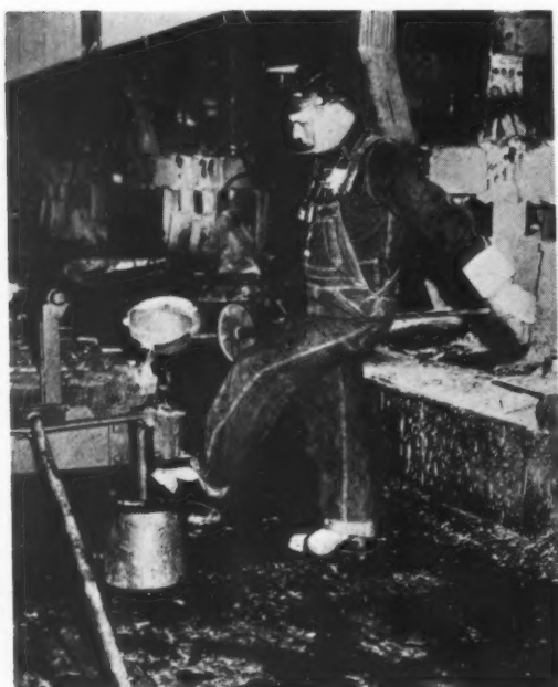
CASTING MAGNESIUM INGOTS AT MIDLAND PLANT OF DOW CHEMICAL, MAKERS OF "DOWMETAL."
