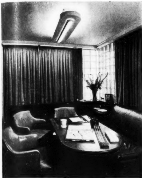
EXPERIMENTAL MODEL OFFICE AT SYLVANIA LIGHTING CENTER ILLUSTRATES MANY DEVICES IN A SMALL AREA. OVERHEAD FLUORESCENT FOLLOWS CONFERENCE TABLE, SHEDS DIRECT AND INDIRECT LIGHT.
