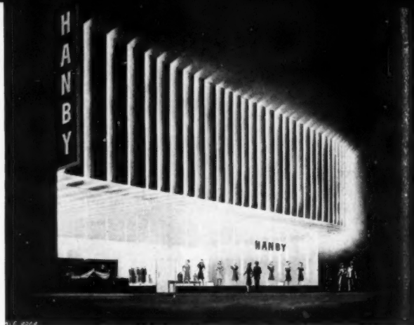
VERTICAL SLIMLINE FLUORESCENT TUBES MEET LINES OF LIGHT RUNNING OUT FROM STORE CEILING. INCANDESCENTS SPOTLIGHT MERCHANDISE DISPLAY. (WESTINGHOUSE)
