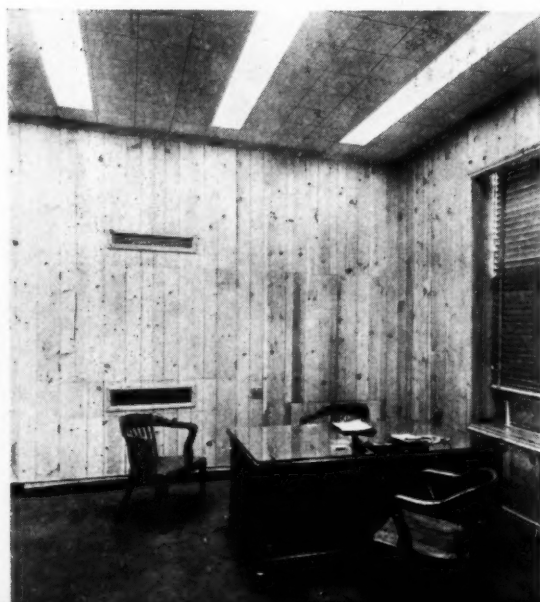
INES OF LIGHT FROM RECESSED FLUORESCENT FIXTURES GIVE EXCELLENT GENERAL ILLUMINATION. HOLOPHANE LENSES DIFFUSE LIGHT IN AN OFFICE.
