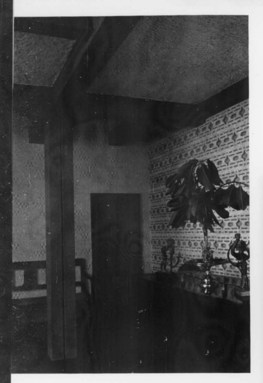
Concrete columns and beams, the existing structural condition which governed Ghika's design, are sometimes chiselled to underscore their massive strength, sometimes furrowed to refine it. Not all the beams are load-bearing—some were added for esthetic discipline.
