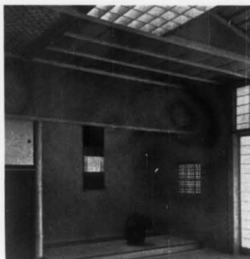
Above: SHINKENCHIKU, No. 8, Tokyo. Complex ceiling design in Japanese room by Sutemi Horiguchi artfully combines various Oriental ceiling types.
