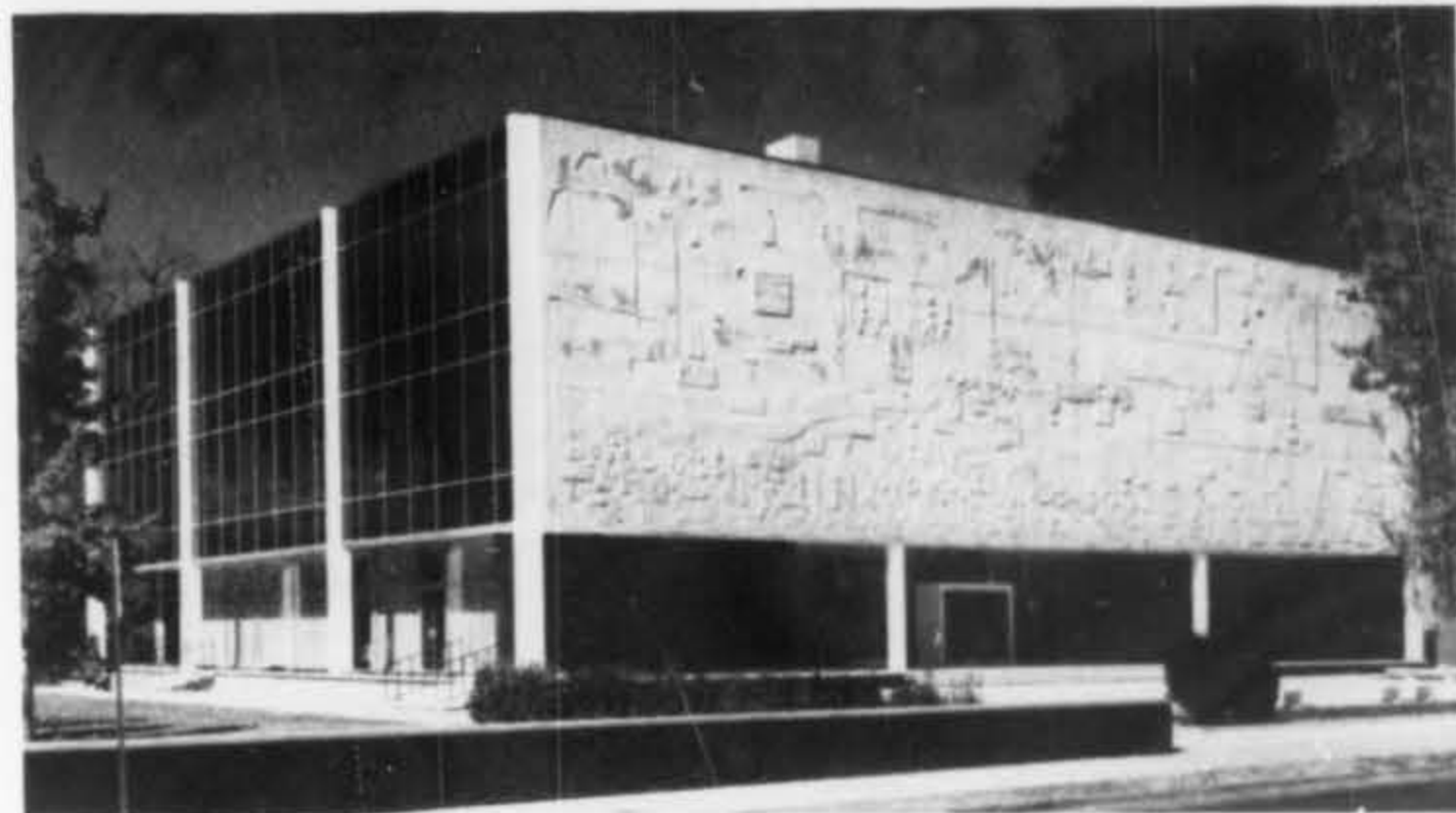
Nivola bas-relief sand sculpture is not an applied decorative ornament but a structural concept at the scale of the architecture. Main floor is set back from building line to create porches on all sides.
