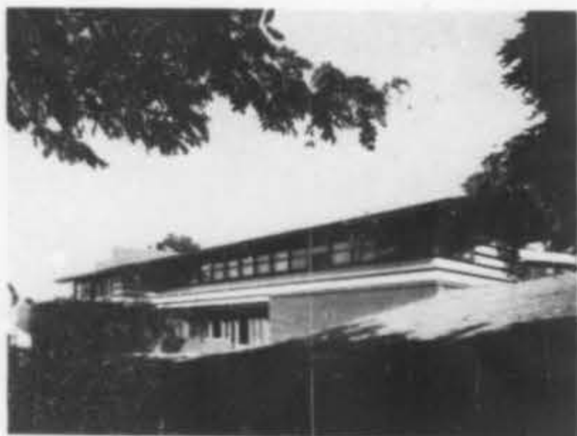
1. Exterior of Frank Lloyd Wright-designed prefab for Marshall Erdman Associates.
