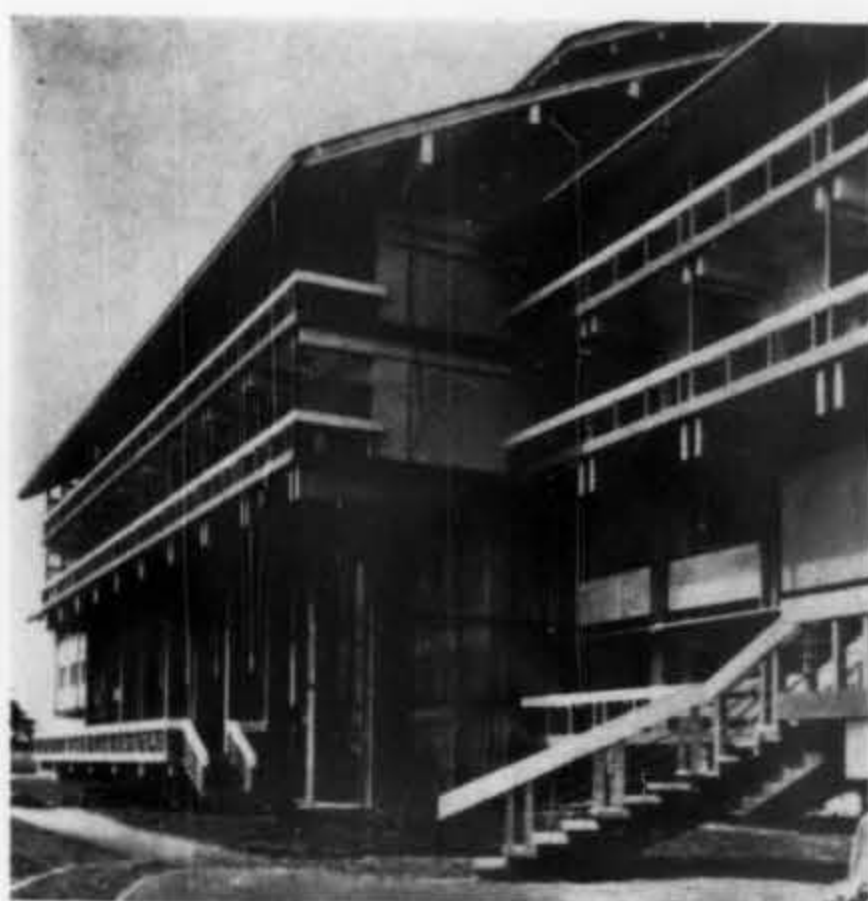
Above: THE JAPAN ARCHITECT, vol. 34, no. 12: The Mt. Hiei Hotel for tourists at Mt. Hiei, Kyoto, by architects Endo and Tomioka; reinforced concrete structure with tiled roof.
