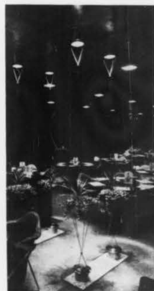
Detail of planters, suspended off floor by taut steel wires, each lighted by a fixture above.
