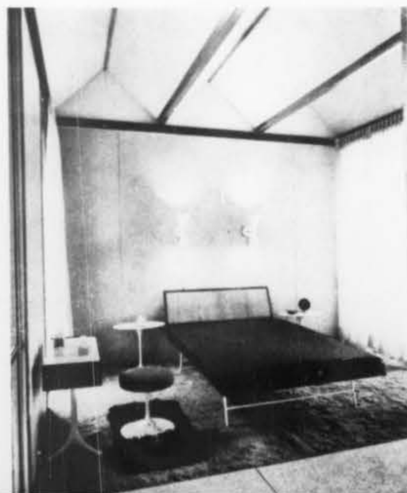
Below: Alcoa House at Milan Triennale. Right: Master bedroom of house showing serrated, folded-plate roof structure.
