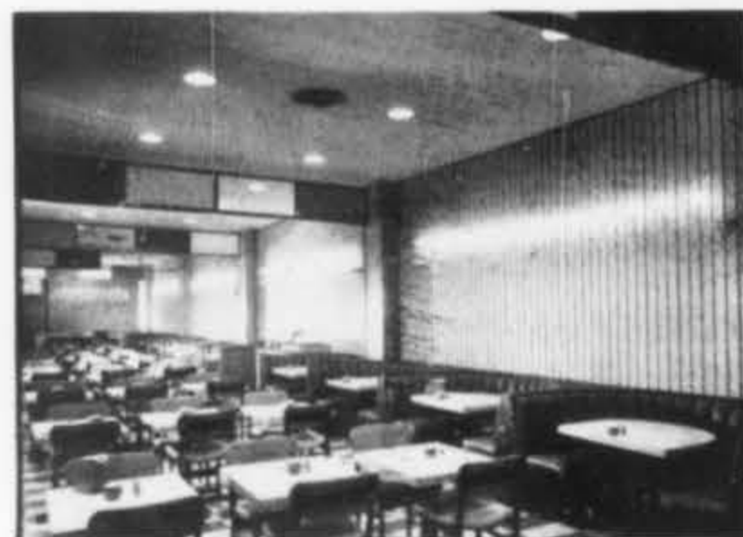
For quick dining, Berliner's Restaurant, Los Angeles, is brisk with smooth materials, high illumination, efficiently handsome geometric design. Wood verticals on a layer of covered fiber glass combine acoustical with decorative treatment. Victor Gruen, architect.
