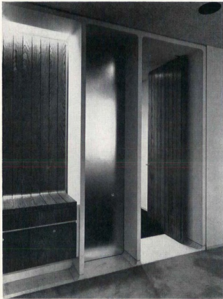
Above: Entrance to an executive office is typical of thoughtful, artistic detailing throughout the job. Planked oak door in the center of a two-foot-deep recess turns on pivots at top and bottom. Terrazzo saddle separates beige rug from deep blue rug inside the office.
